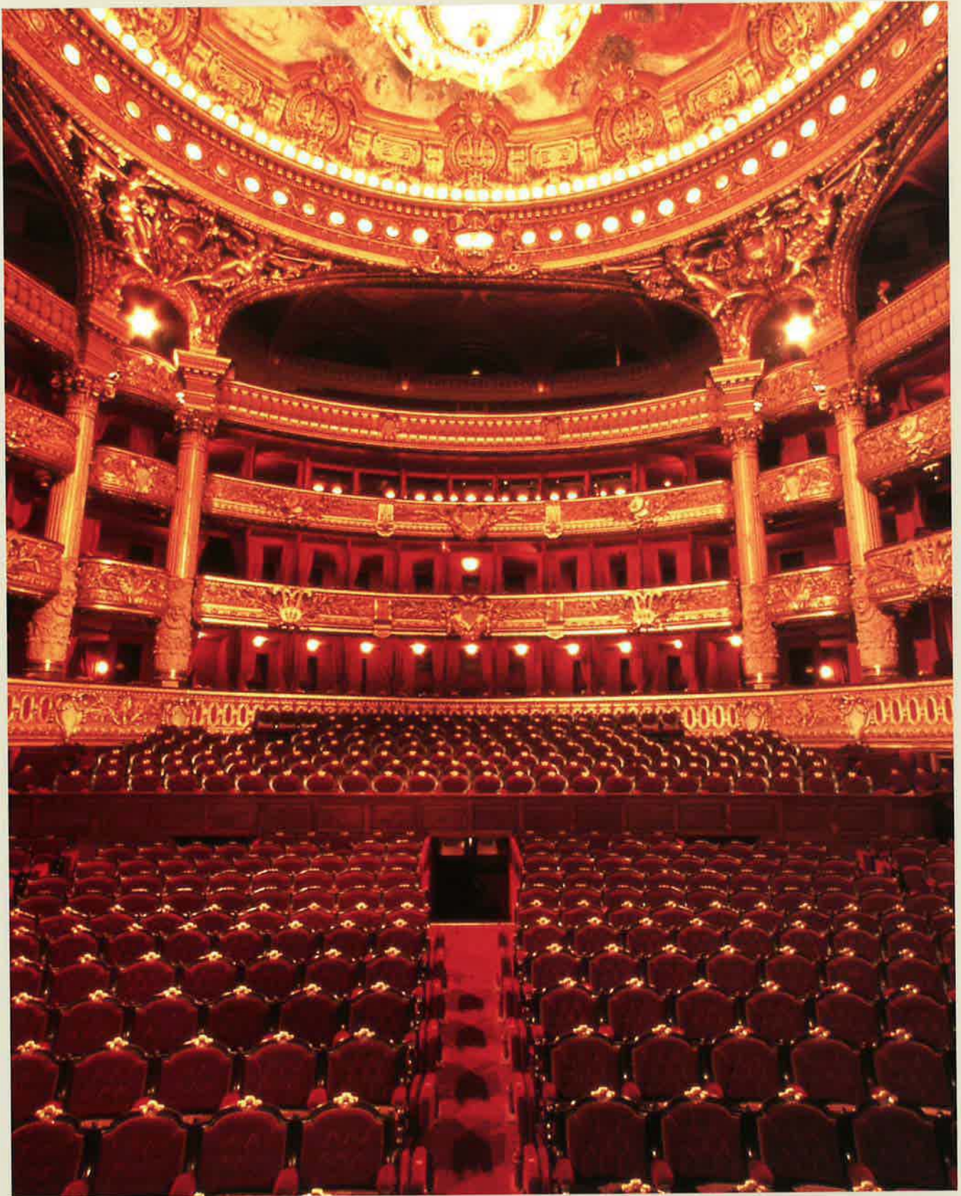
SDEL took part in renovating the main hall and the electrical systems of the Opéra Garnier, which reopened on 1 March 1996 after two years of work.
