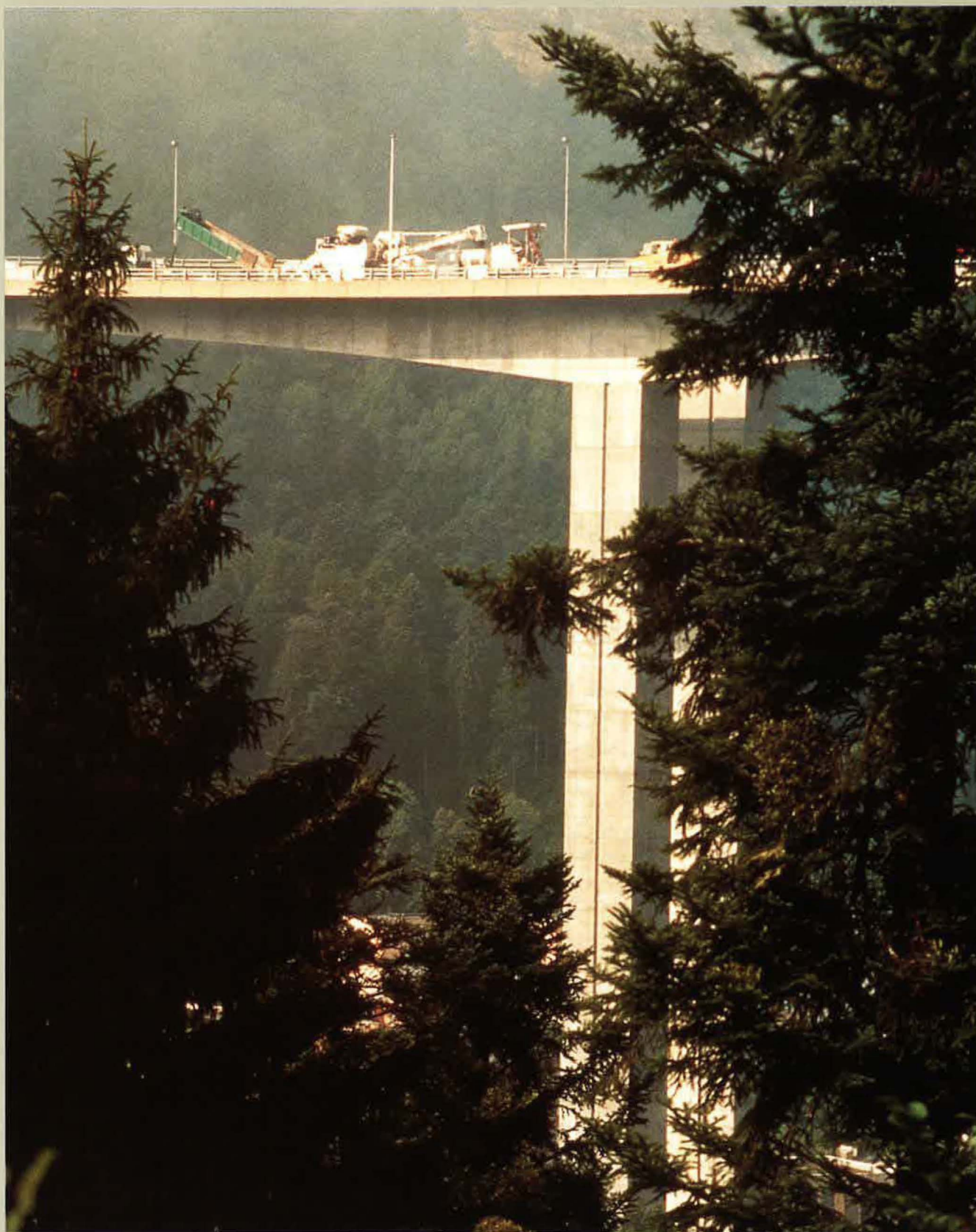
Viafrance paved the roadways of the new Nantua and Neyrolles viaducts on the A40 motorway (Mâcon to Geneva to Chamonix).
