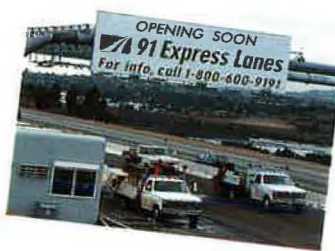
Since late 1995 Cofiroute has been operating a 16 km toll road built along the median of the SR91 highway in southern California. The new road serves San Bernardino, Orange, and Riverside counties near Los Angeles and is available only to motorists using an electronic toll system.
