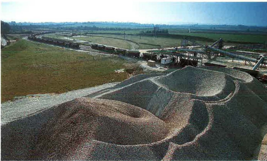
Acquired by Viafrance in 1989, the Chailloué quarry in Orne doubled its output in order to supply aggregates for the A29 motorway, to be built between Le Havre and Yvetot.
