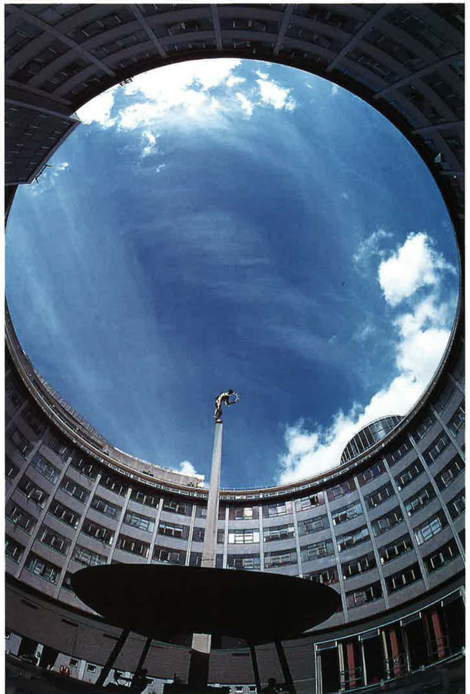
Norwest Holst remodeled an old television studio in London's West End to serve as the BBC's new head office.
