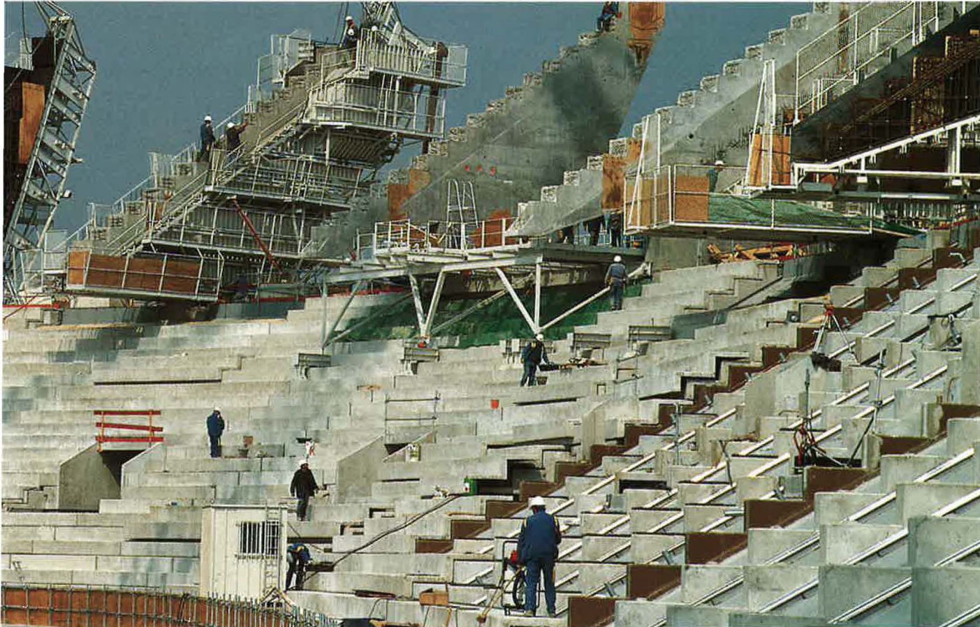
The cornerstone for the new Stade de France was laid on 6 September 1995. Six months later, more than half of the rough work was completed, with the foundations finished and the intermediate seating tiers in place.
