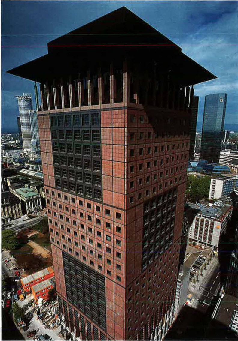
Heinrich Nickel installed the air conditioning for the Japan Center tower, under construction in the business district of Frankfurt-on-Main (Hesse).
