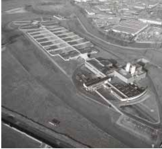
The Beaurade purification plant near Rennes has a capacity of 350,000 population equivalent. It was opened in June 1997.
