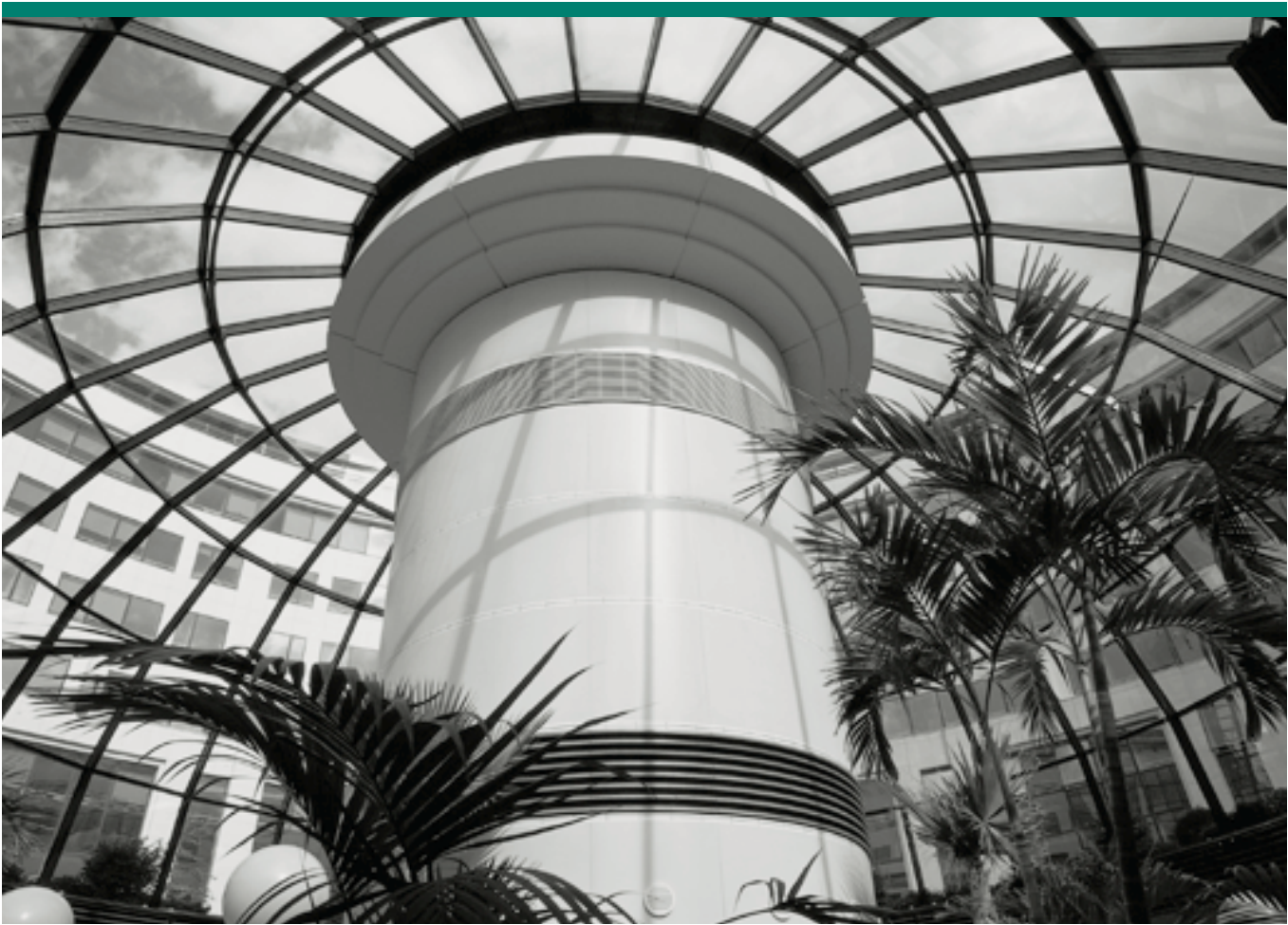
Lefort Francheteau supplied the air conditioning for several buildings – including the Arte television channel headquarters – in Issy-les-Moulineaux, just outside Paris.
