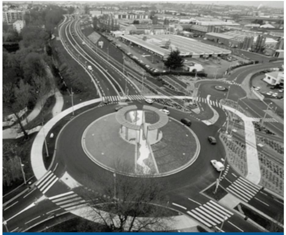
Eurovia builds roads, roundabouts and urban thoroughfares in large and small towns.
