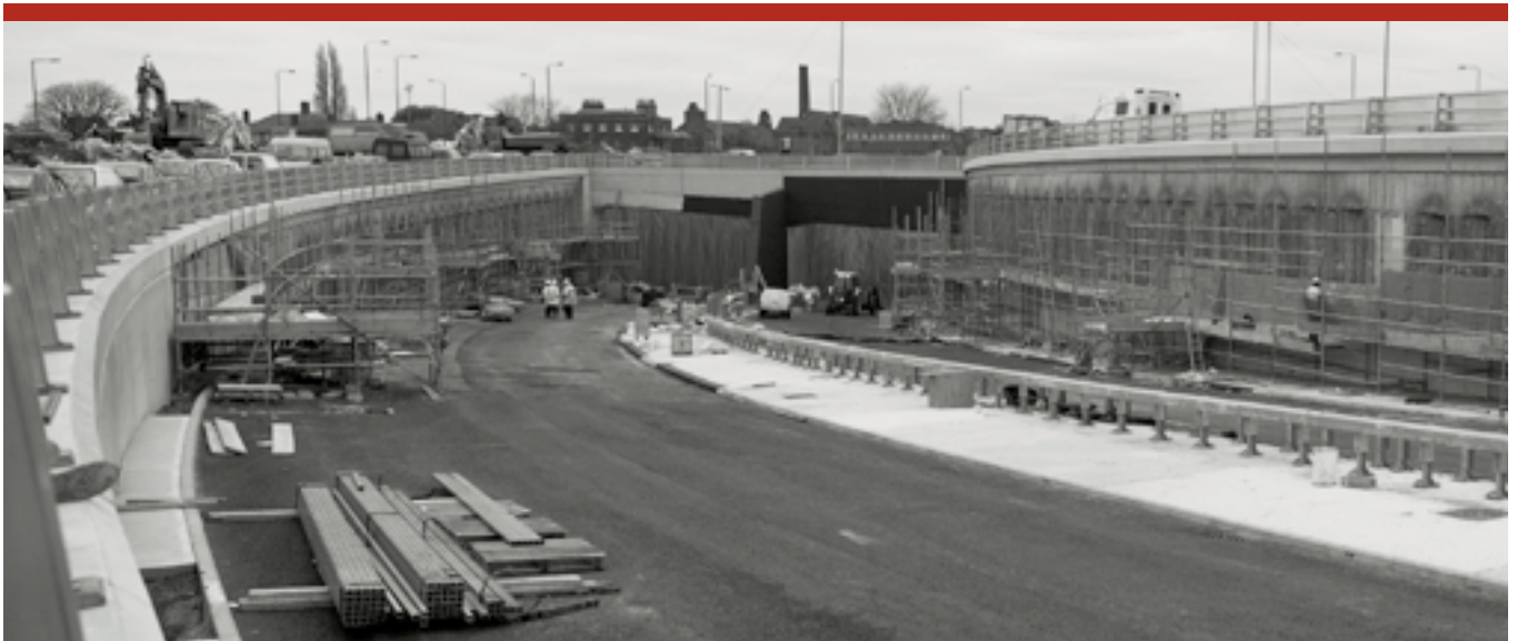
Civil engineering work on the A12-M11 link road east of London.
