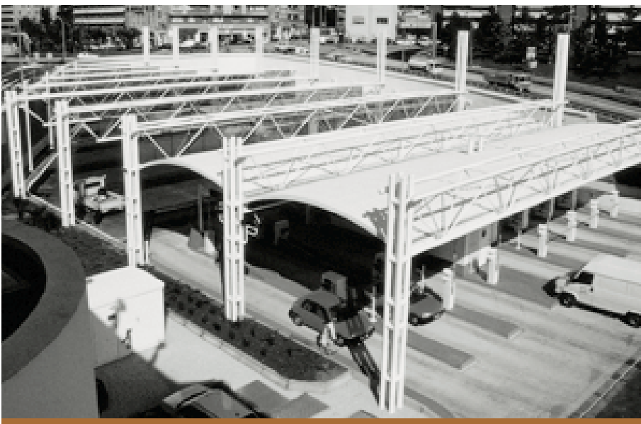
The Prado-Carénage tunnel has provided an underground crossing for Marseilles since 1993.
