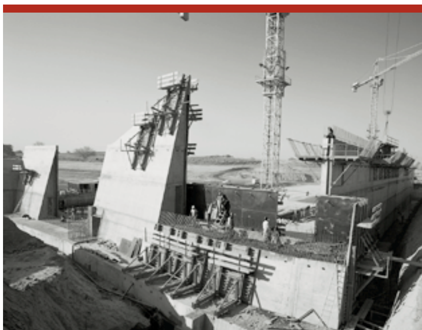
Building the Ziga dam of compacted rolled concrete in Burkina Faso.
