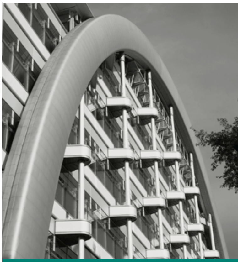
G+H Montage provided the façade and roof surfacing for the new Tatou building, designed by architect Nicholas Grimshaw, where the Berlin stock market will be housed.
