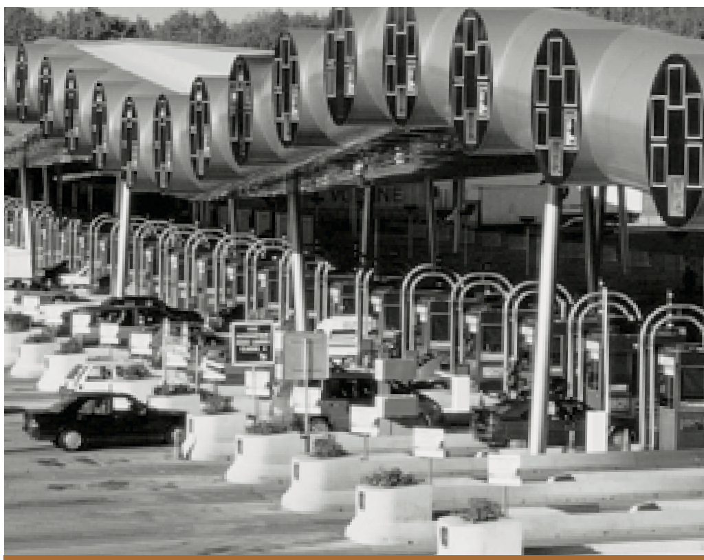
Cofiroute, the world's leading private motorway concession company, operates some 800 kilometres of motorway in France.
