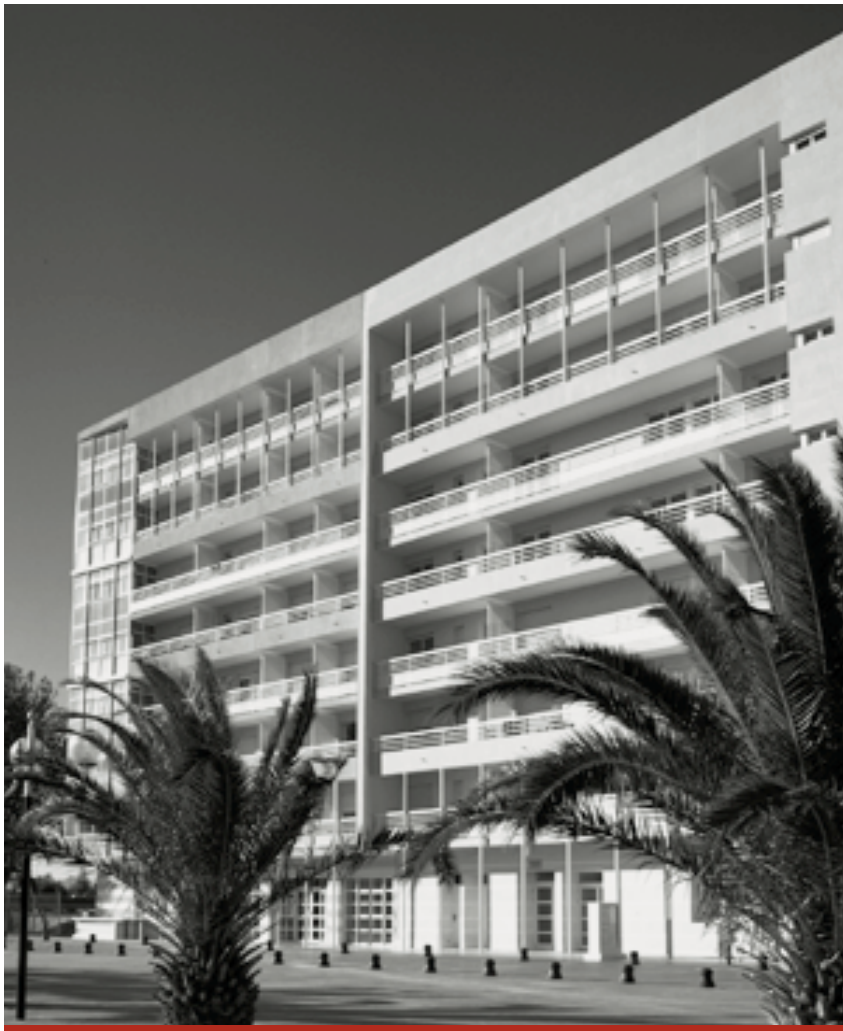
Sogea, as general contractor for the Caisse d'Epargne property group, built the 56 studio apartments of the Universalis 2 students' residence in Perpignan, in the south-west of France.
