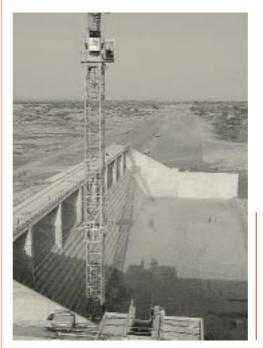
Sogea has a very tight deadline to complete the Ziga barrage in Burkina Faso. A main feature of the project is its use of a special type of compacted cast concrete. In all, 36,000 cu. metres of concrete will be used.
