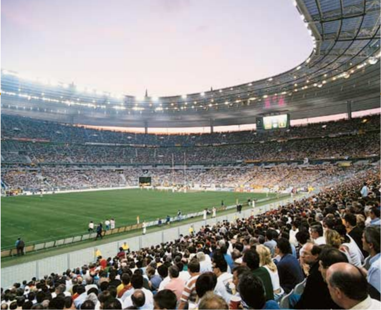
The Stade de France, offering seating capacity for 80,000, has been the venue for a wide range of sporting and cultural events, which were mostly sell-outs.
