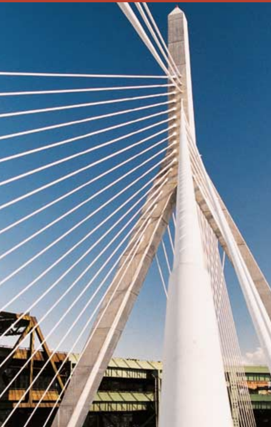
The Charles River bridge in Boston, where Freyssinet supplied the cable-staying. With a width of 56 metres, a world record for this type of bridge, it will carry ten lanes to ease the flow of traffic.
