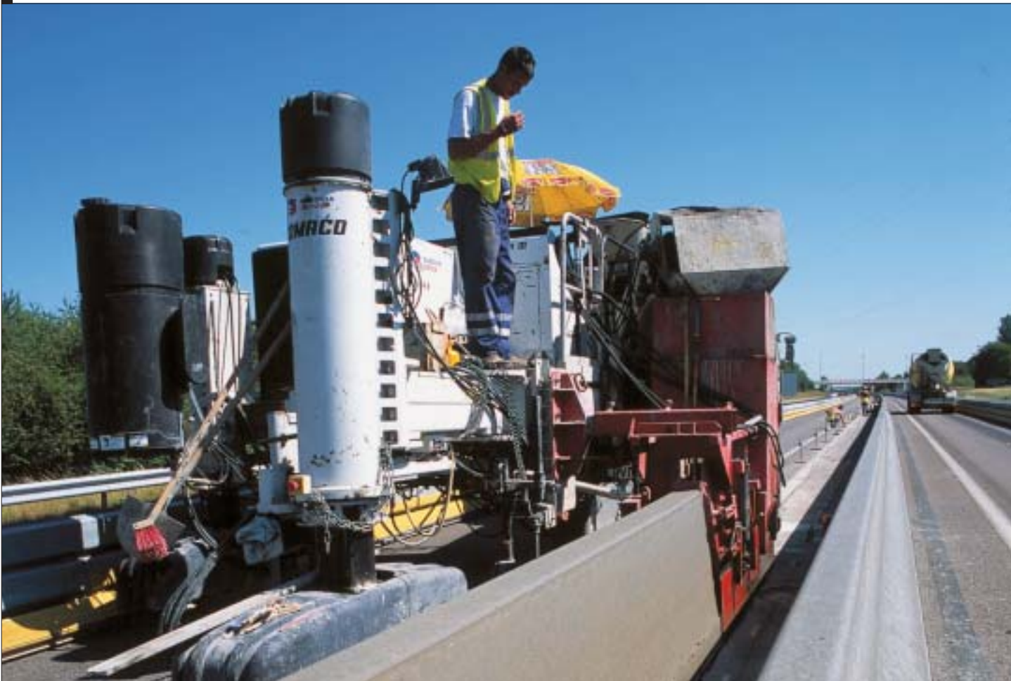
Installation of concrete separators on the A6 near Beaune, France
