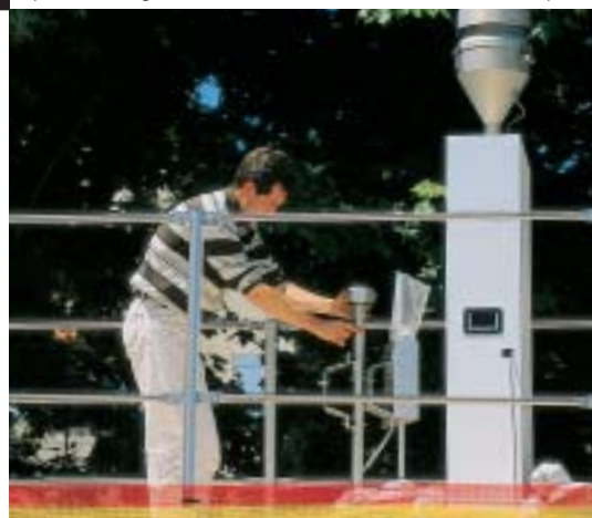
VINCI Energies designs and implements environmental monitoring systems throughout the world for local authorities and industry
