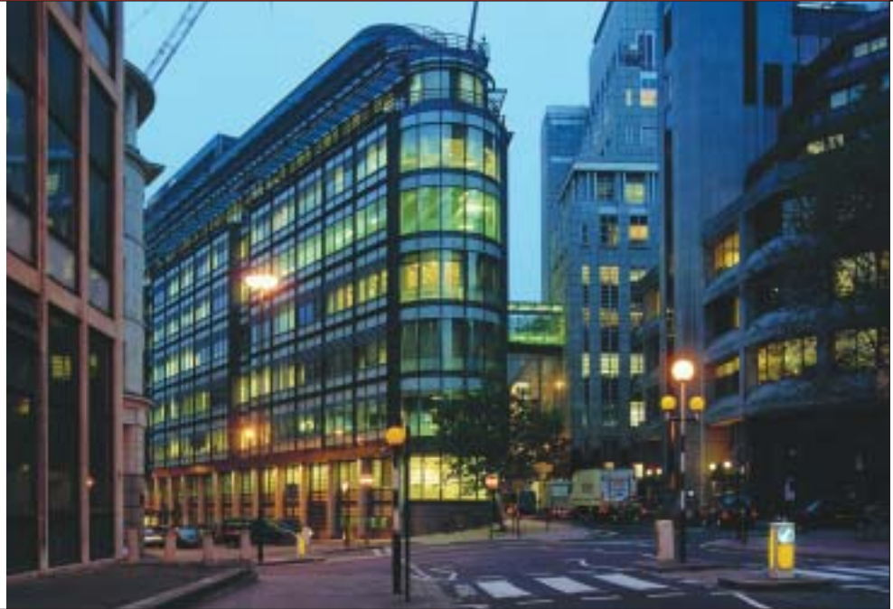
Renovation of a 27,000 square metre office building in central London
