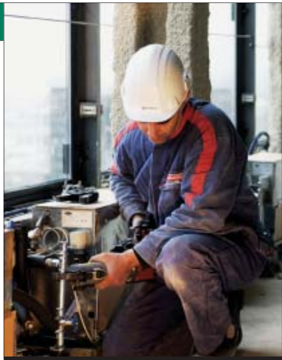
Installation of air conditioning at the Nobel Tower in Paris-La Défense
