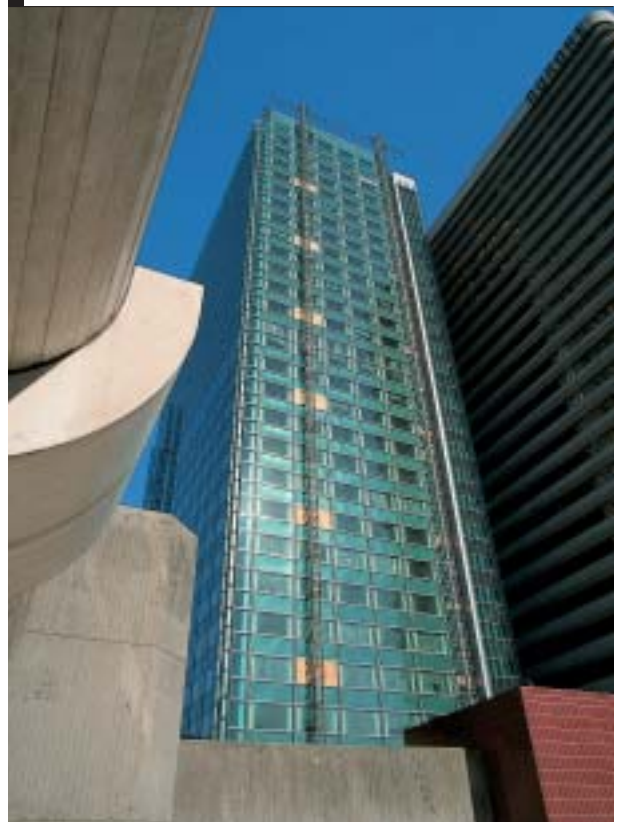
Structural rehabilitation of the 28 floors and 6 underground levels of the CB16 tower in Paris's La Défense business district
