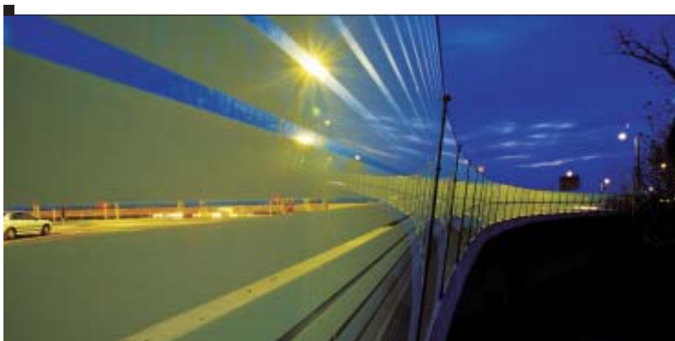
The 1,000 metre noise-abatement wall on the new 2 x 2-lane 10 km section linking the A9 motorway to the gates of Leipzig
