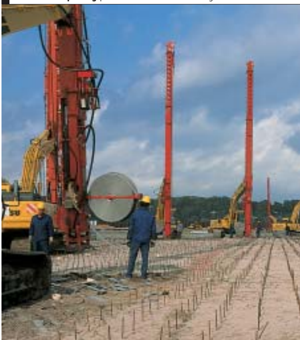
Vacuum compacting prevents the soil from settling ■
