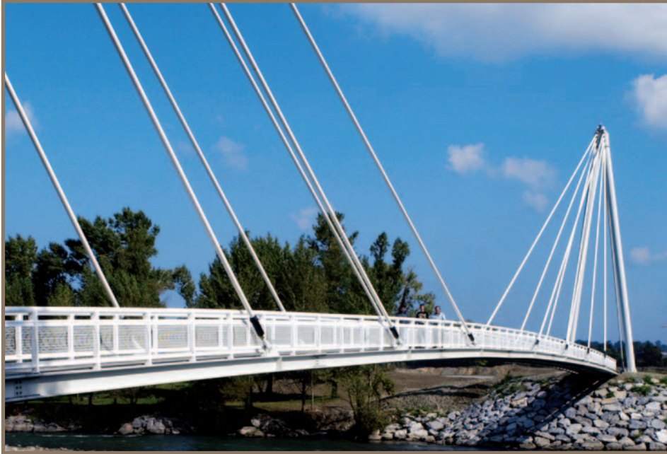
Freyssinet won FNTP's (the French Federation of Civil Engineering) top innovation prize for carbon fibre cables. Used for the first time on the Laroin footbridge in France, the cables help improve a structure's durability.
