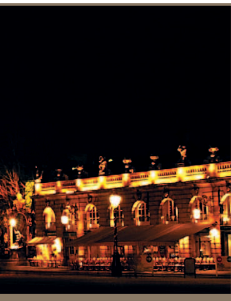
Public lighting and landmark enhancement in Nancy, France.
