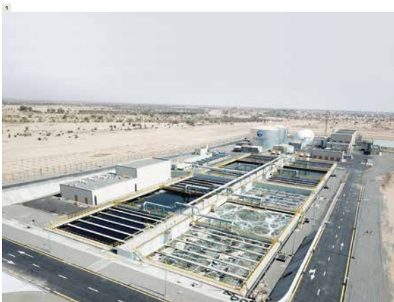
1 Construction of a wastewater treatment plant in Saudi Arabia with capacity of 100,000 cu. metres/day, expandable to 270,000 cu. metres.
