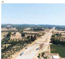
1 The Athens–Corinth–Patras motorway concession adds a new 75 km section linking it to the city of Pyrgos.
