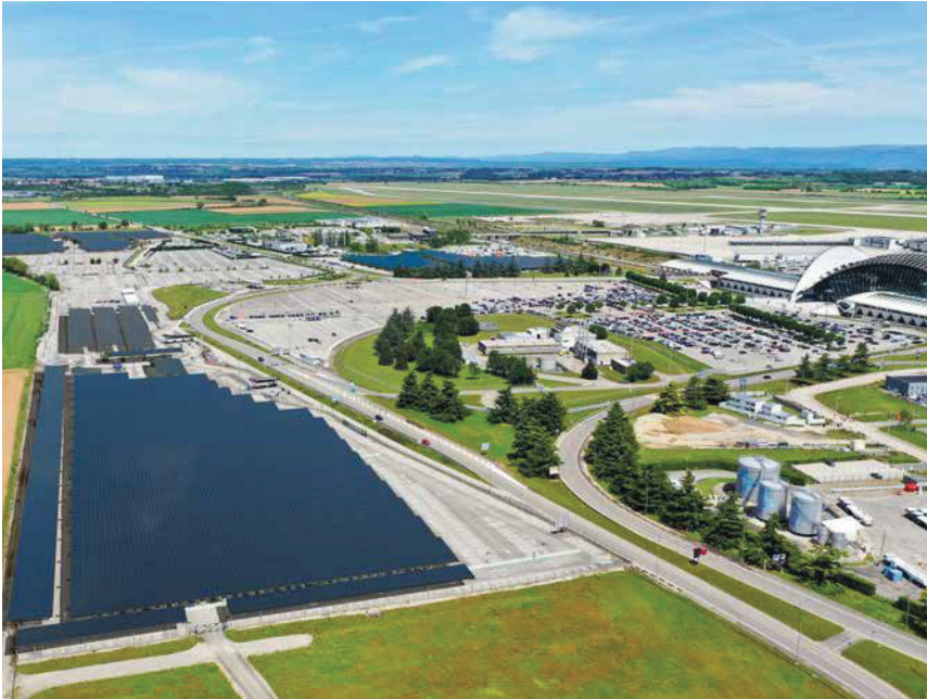
At Lyon-Saint Exupéry airport, the VINCI Concessions subsidiary SunMind partnered with Neoen to deploy one of France's largest solar canopies, spanning 14 hectares, with a capacity of 20 MWp (computer-generated image).
