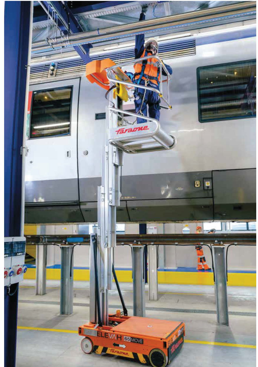
Actemium's teams carry out maintenance at 14 of SNCF's technical centres (France).
