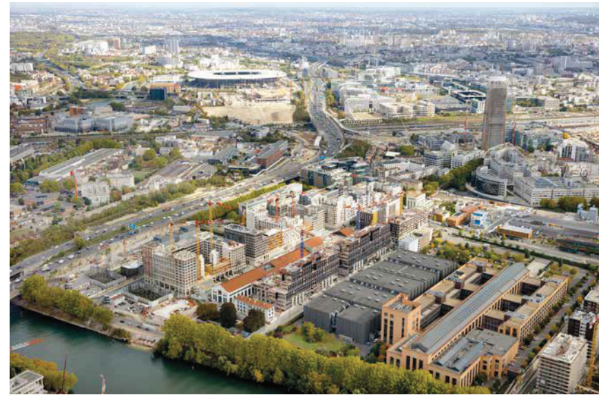
With the Athletes' Village, extension of metro Line 14 to the north and the Saint-Denis Pleyel terminal, redesign of the Pleyel/A86 interchange system and other projects, all of VINCI Construction's business units are working together to play their part in ensuring the success of the Paris 2024 Olympic and Paralympic Games in and around Universeine.
