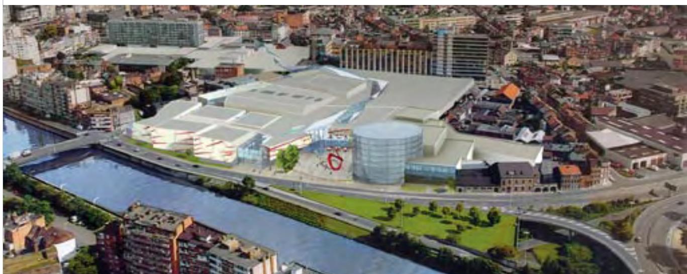
"Médiacité" business complex at Liège. Architect: M. & J.M. Jaspers - J. Eyers and Partners. Developer: Withem & C° - BPI.
