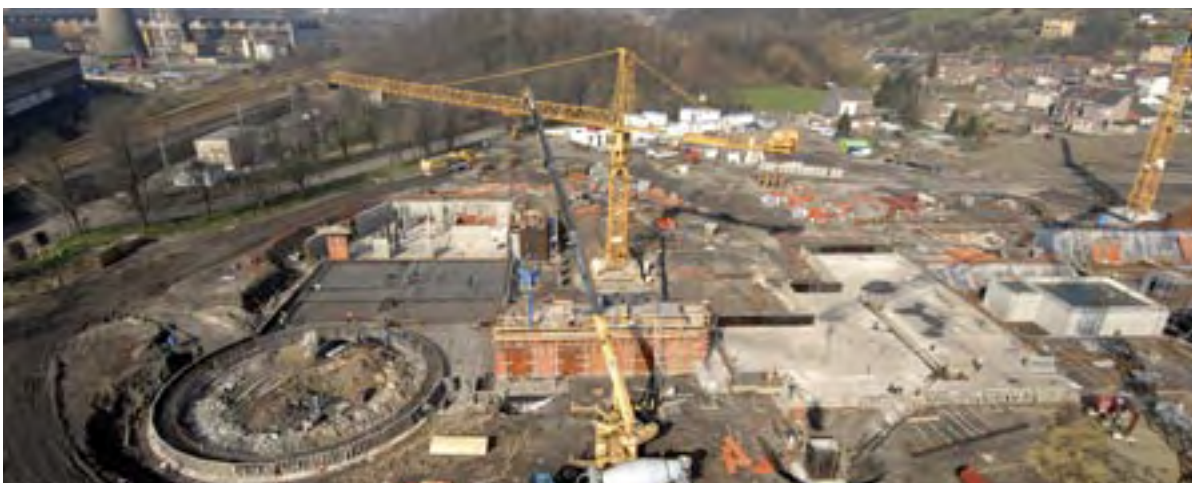
The water-treatment plant at Liège - Sclessin. Architect: Daniel Lesage.
