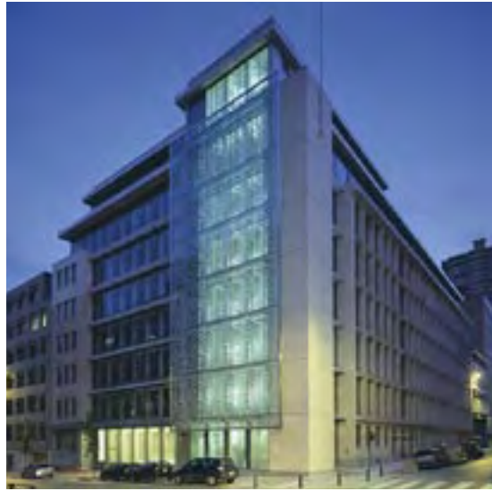
"Montoyer" building in Brussels. Architect: Assar - Mr Ysebrant et Mr Morales.
