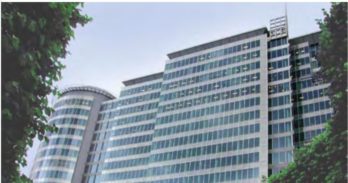
"Botanic" building in Brussels, managed on behalf of Crédit Suisse. Architect: A.M. L'atelier d'architectures de Genval - Pierre Accarain SA - Marc Bouillot SA.
