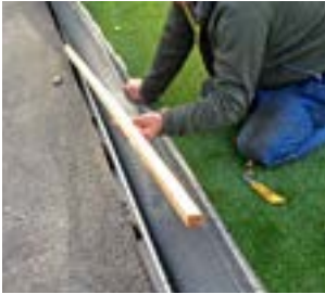
Removing the cistance elements (to be disposed of by the customer).
