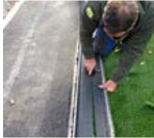
The artificial turf is cut to the right length.
