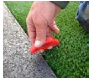
The fastener is turned over the curve by 90 ° and the installation key pulled out.
