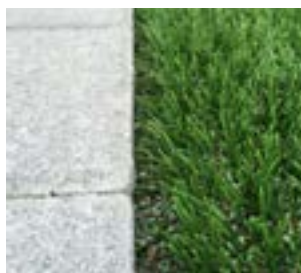
Paving stones / artificial turf (The artificial turf closing elements, which are set lower than the paving stones, are not visible).
