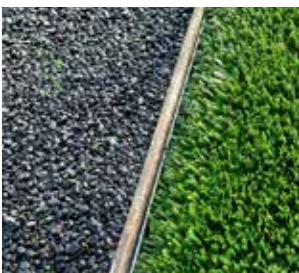
Covering / artificial turf (in order to increase the surface area a metal strip (flat steel) was used here).
