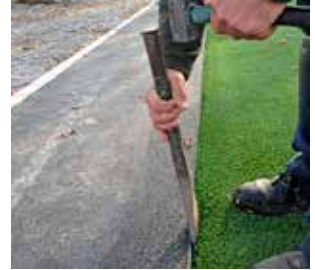
For thick or high-pile artificial turf aids such as seated iron can be used.
