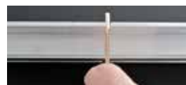
The necessary gap of 2 mm (material expansion) can be ensured with a match.
