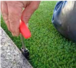
The fixing element is inserted into the installation element by means of the installation key, down to the lower web (note the pictures on the previous pages).
