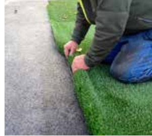
The artificial grass is pressed into the installation element.
