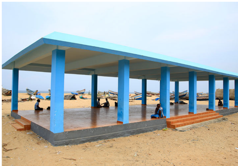
Fig 10.7: Permissible Open structures for fishery related activities between 200 and 500 meters above the HTL
