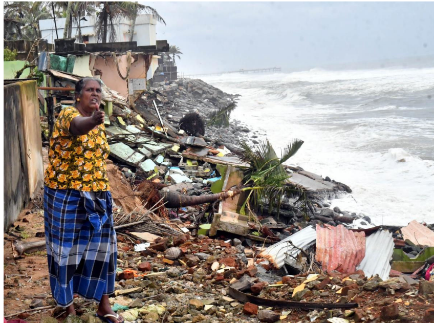
Fig 7.2: Shangumukham Beach Road in 2021 impacted by coastal erosion north of the VIS (Valiyathura Pier in the background)
