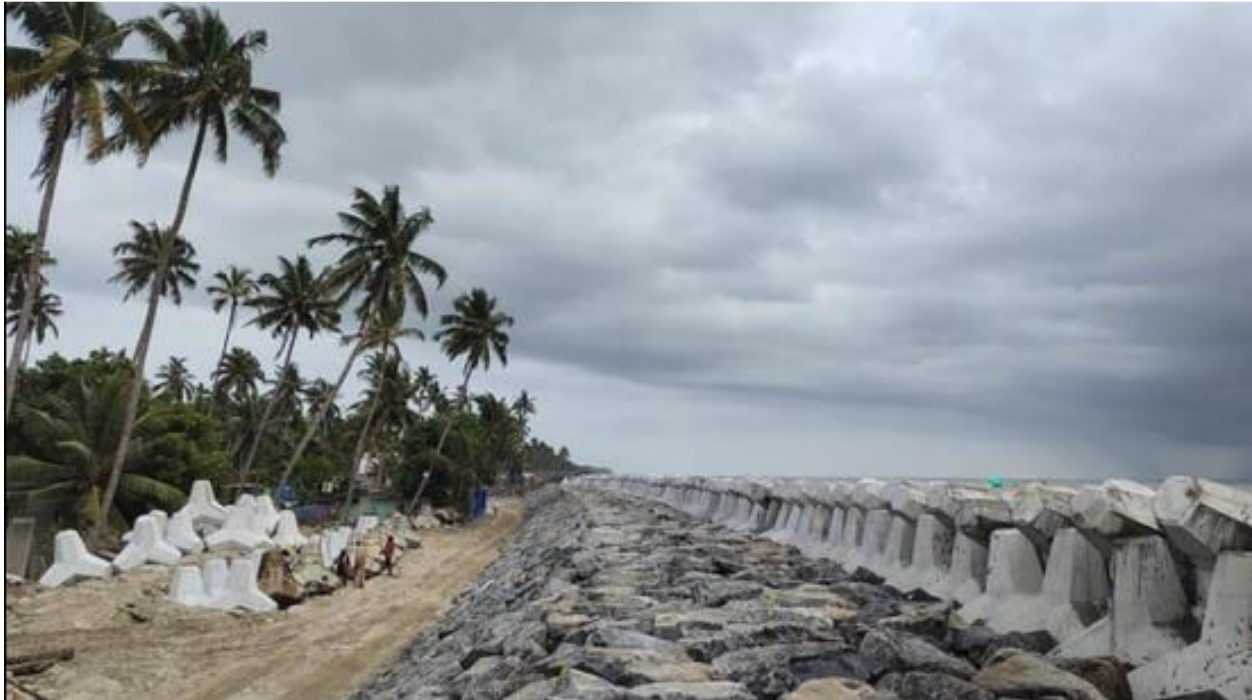
Fig 10.1: Seawalls of Chellam (2022): Perhaps a coastal engineering marvel, but an ugly eyesore and not a solution
