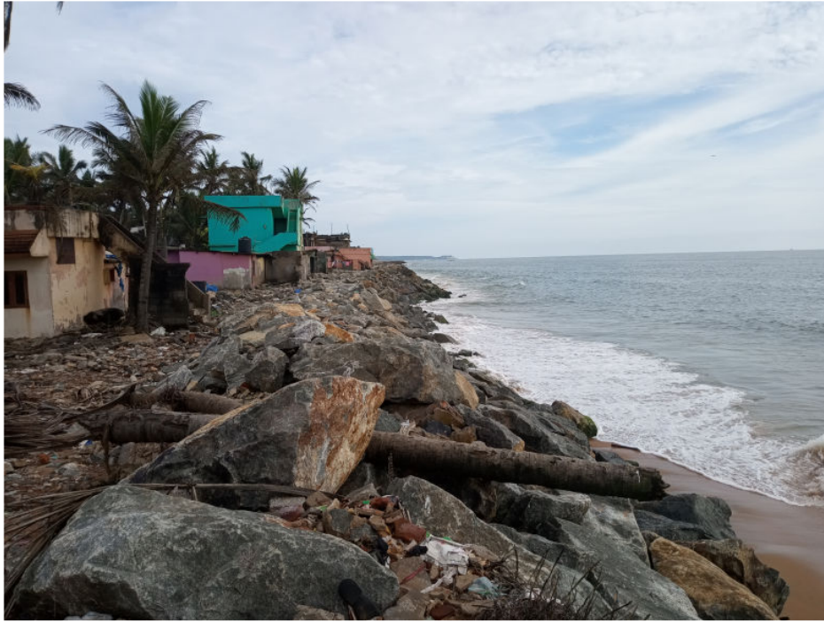
Fig.5.20. Valiyathura – south of pier (March 2018)
