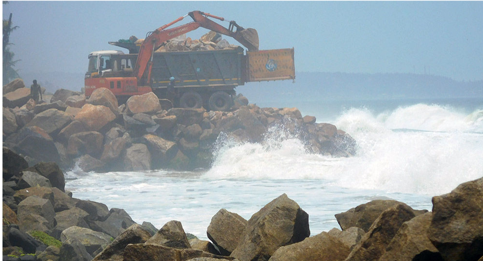
Groyne construction in progress in Valiyathura.
