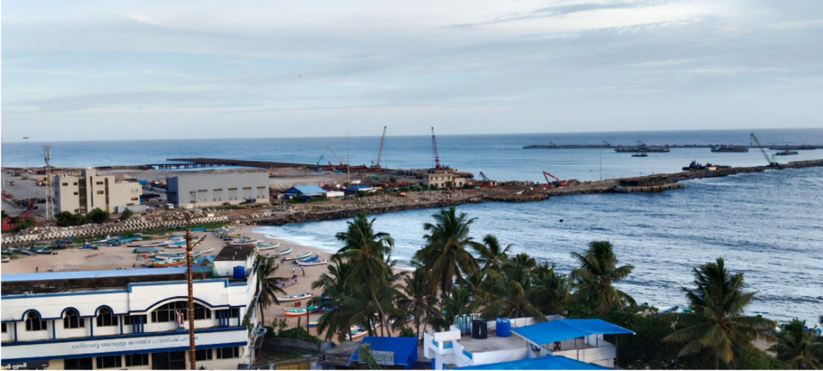
Fig 11.1: VIS Breakwater as on June 3, 2023
