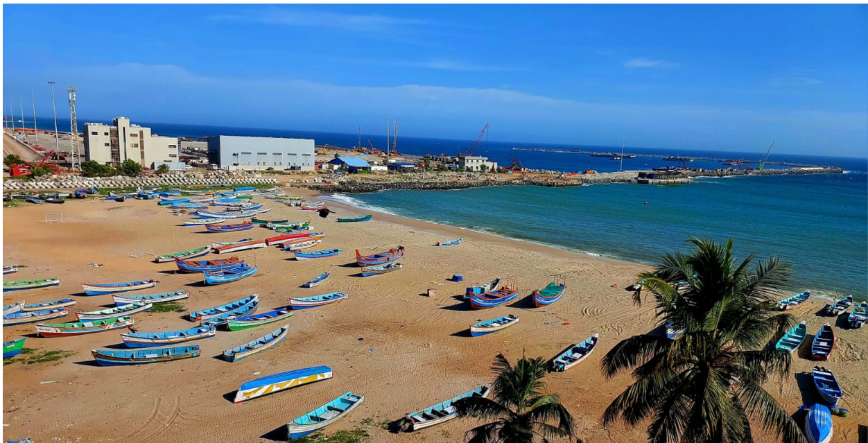
Fig 5.22: Substantial beach building observed at Valiya kadapuram adjoining to and between the harbour mouth and the port breakwater under construction Credit: Probir Banerjee
