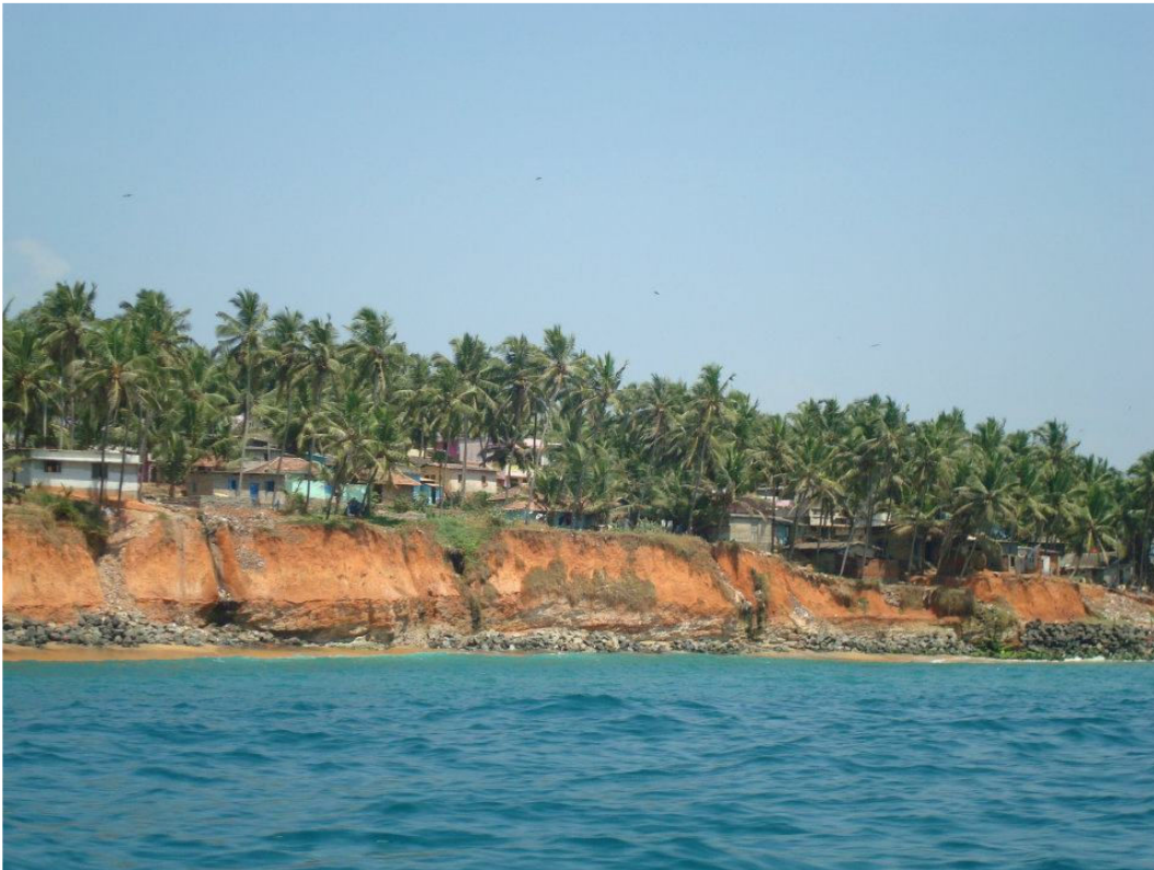
Fig. 5.17. Eroding cliffs (photo of 2013) south of Vizhinjam Fishing harbour and close to the VIS site – Still the EIA claimed Vizhinjam and adjoining coasts as stable (Photo of 2013; Credit: Cyriac Kodoth)
