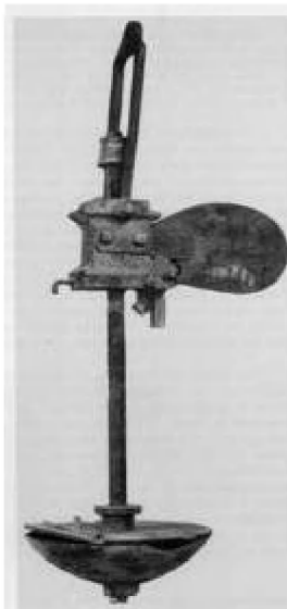
Figure 4. Detail of the ground-collector. Source: Carpine, 1996
