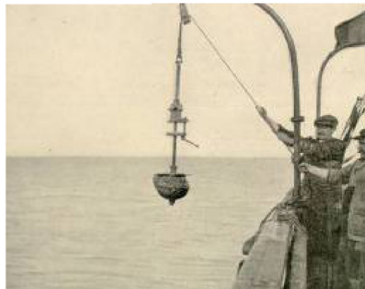
Figure 5 . The ground-collector, over-filled with mud, is hauled onboard (source: Gilson, 1927)
