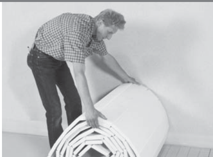
Unroll and lay out the Stapler system elements.
