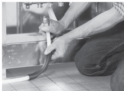
Attach the heating pipe to the manifold and you're done!
