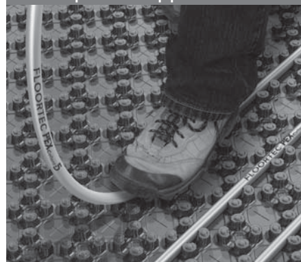
Fig. 1: Laying of Pe-Xcellent 5 underfloor heating pipe
