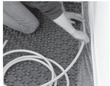
Figure 2: Fixing the additional strip of film
