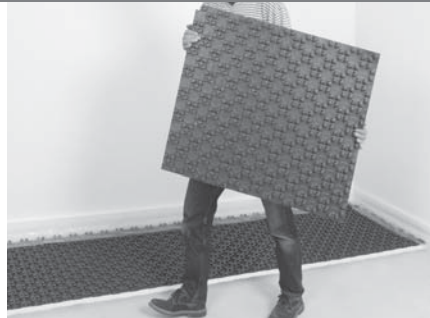
Lay the plates from left to right.
