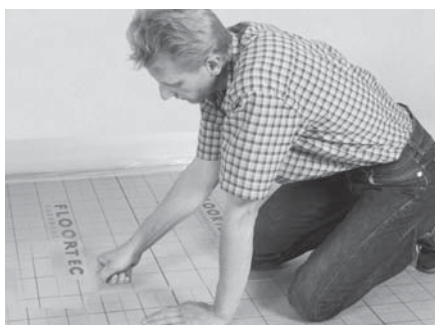
The rolls of insulation include a 3-cm self-adhesive strip and overlap at the joints.
