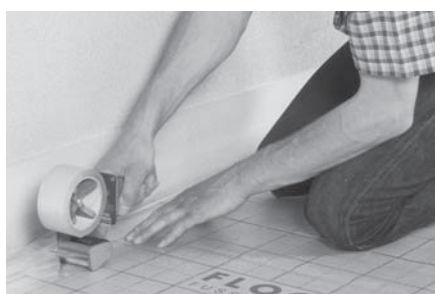
Figure 6: Sealing down the film apron
