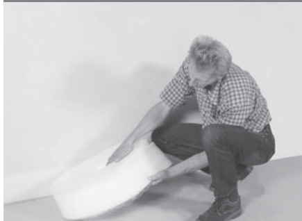
Install the edge insulation strip with its attached film apron.
