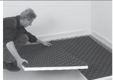
Continue laying the FLOORTEC System Preformed Plates.
