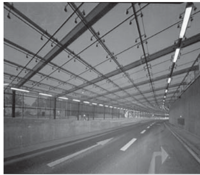
Petuel tunnel in Munich, Germany
