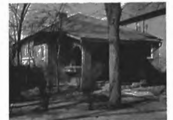
FORMER LIBRARY HOME 508 Park Avenue
