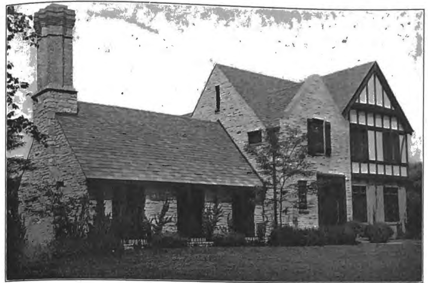
Administration Building, Cook County Forest Preserve, Cummings Square, River Forest.
