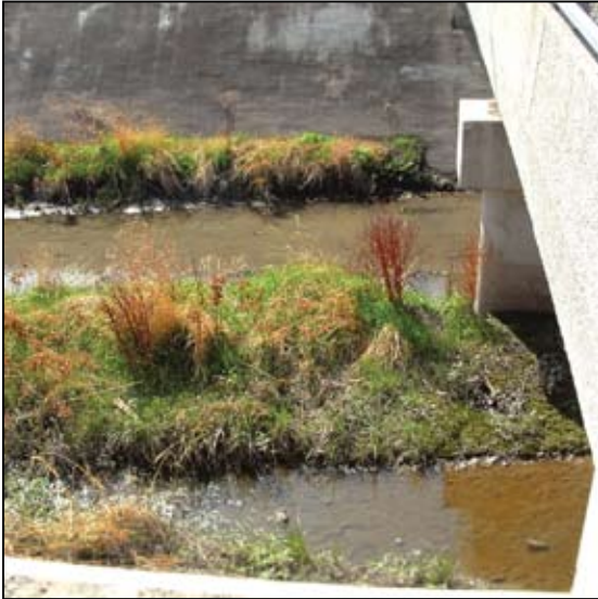
Berryessa Creek west of railroad corridor looking north
