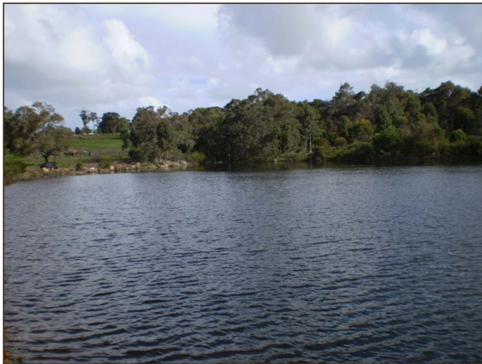
Plate 2: Looking south-west across the main dam from the dam wall.
