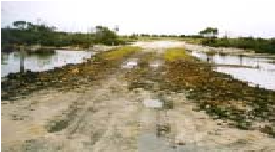
Crossing on Sue and Peter Smithson's property. This is an excellent example of a crossing as it has many small and varied sized rocks, follows the contours of the river and is located in a relatively straight section of the waterway. This design is recommended, as it is more likely to survive flood events and cause less erosion and sedimentation. The rocks cause the water to trickle downstream adding oxygen to the water that is important for aquatic fauna (photograph Kaylene Parker, WRC).
