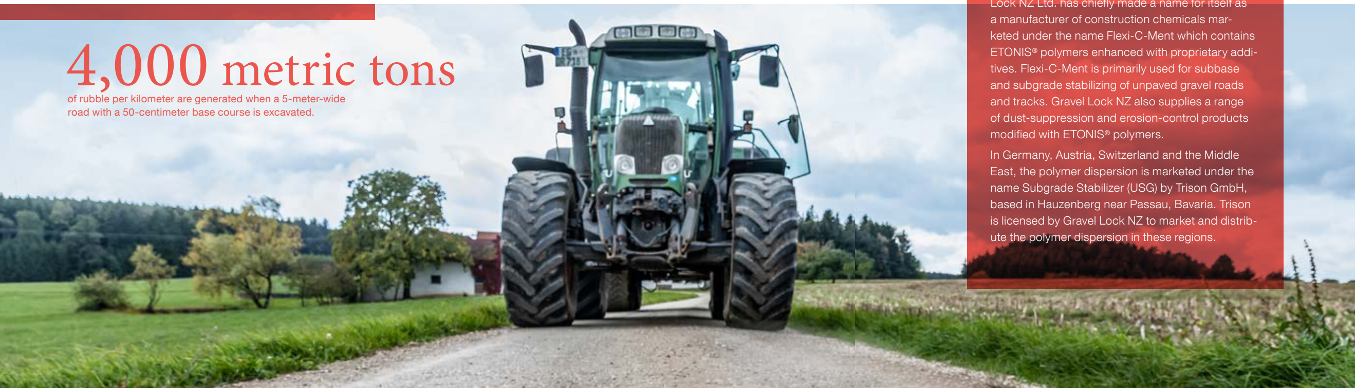
In the hamlet of Hebertsfelden in Bavaria, a farm track leading to a farm was treated with a subgrade stabilizer. The test section shows that a structure strengthened in this way can withstand high loads undamaged.
