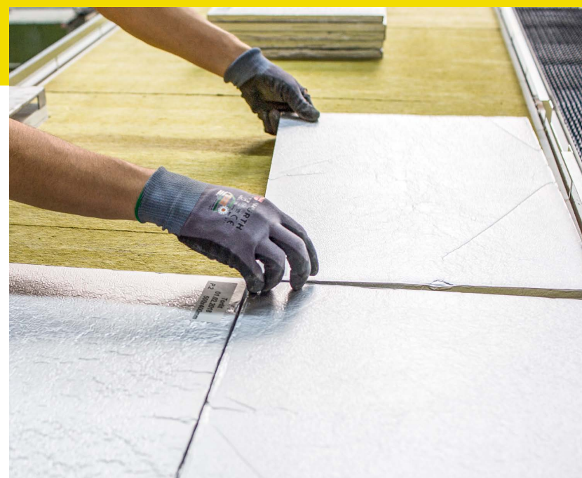
If vacuum insulation panels are intended for use on a construction site, Vitec customizes them and automatically supplies the installation plans as well.
