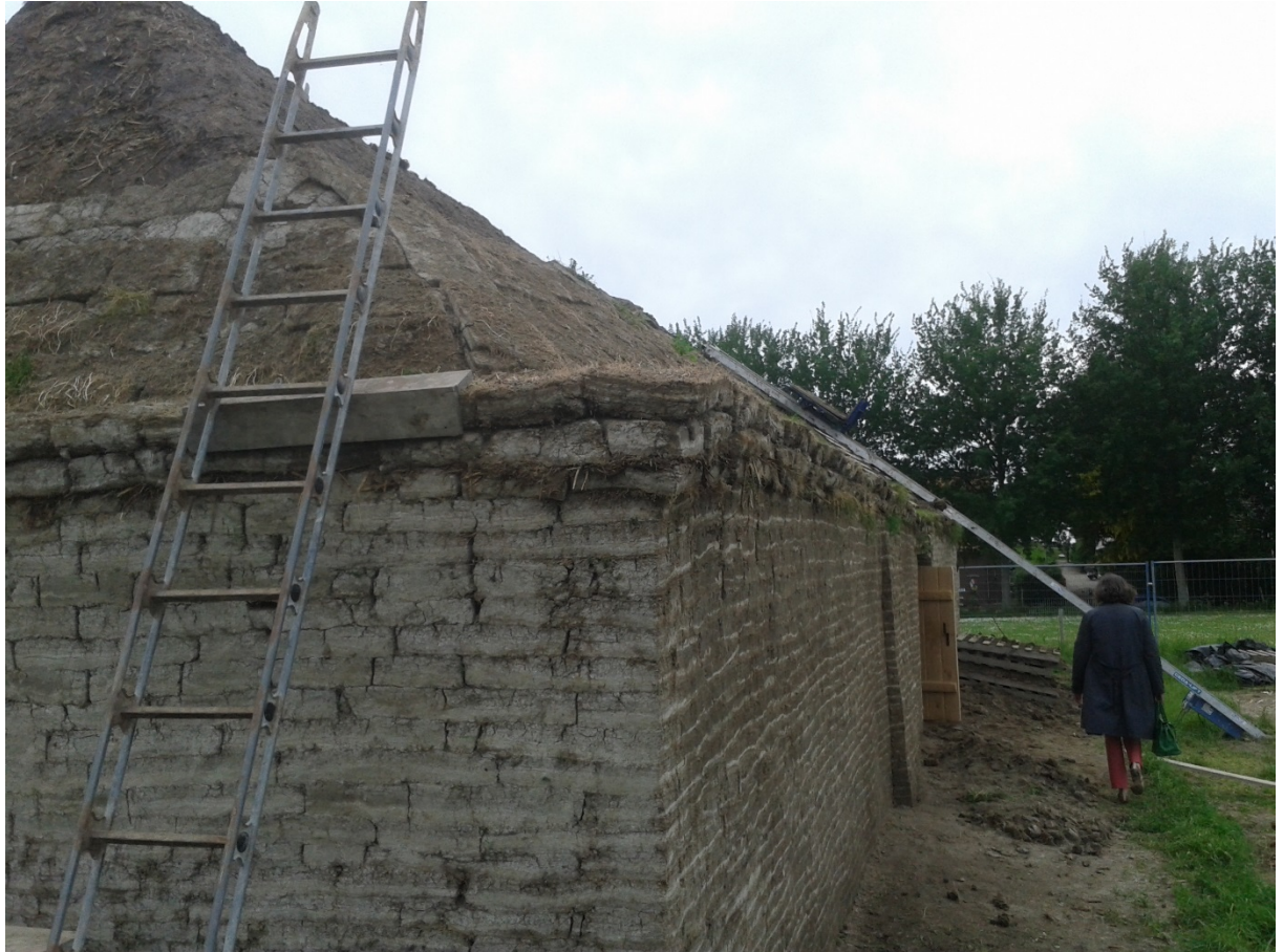
Reconstruction of a sod-house in Firdgum (Fryslân). The first settlers on the mainland Wadden coasts, induced by lack of building materials, probably built their houses by means of sods dug in the salt-marshes (photo: Meindert Schroor)
