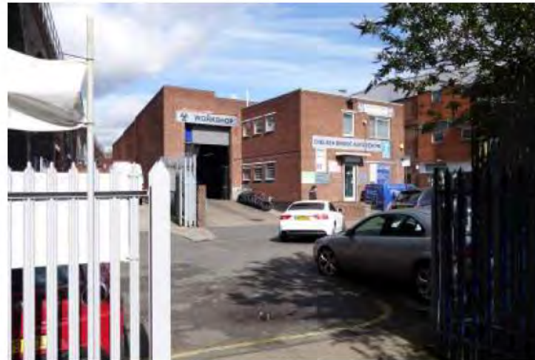
02 - View of MOT Services opposite the site
