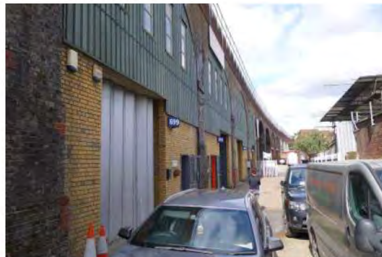
03 - View North from within the Network Rail access road (Site to right)
