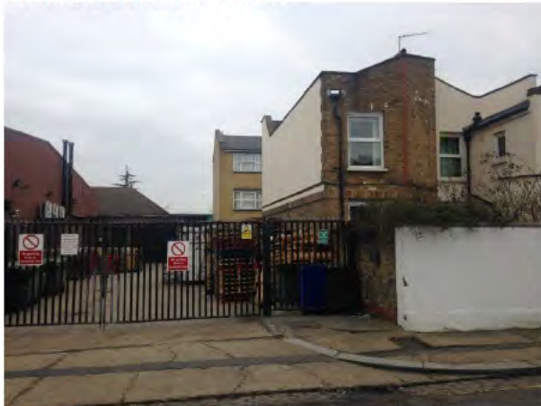
Rear of residential properties within the LSIA
