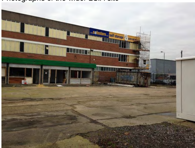
Former Europcar and Safestore site (currently being demolished)
