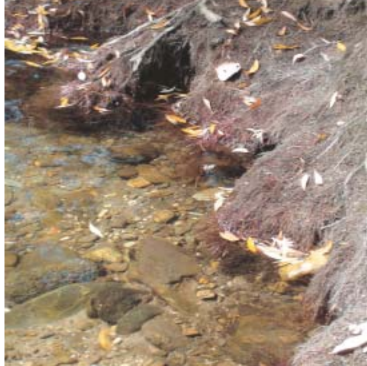
Fluvial scour underneath a willow root mat. Photo Lizzie Pope.
