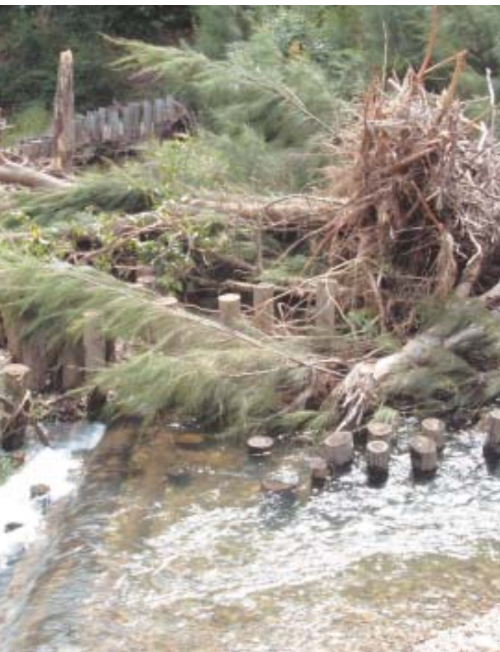
Elevated log sill structure has trapped flood debris that will later provide valuable habitat. Photo Andrew Brooks.
