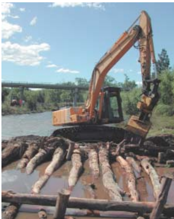
Left: Constructing a log jam. Right: Stream with hydraulic changes as a result of wood reintroduction. Both photos Dan Keating.
