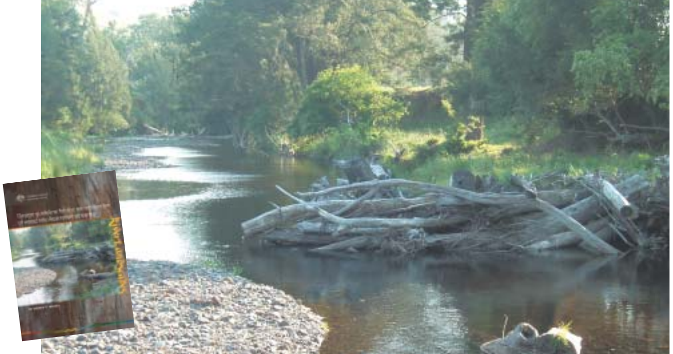
River rehabilitation using an engineered log jam. Photo Tim Howell.
