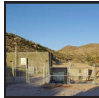
Municipal water source/ water treatment plant
