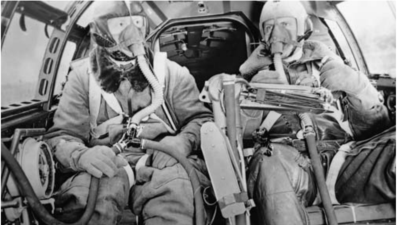
1943 High altitude breathing apparatus for military aircraft. ▲
