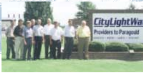
The Paragould gas power plant was delivered to the customer in June. The power plant is located in Arkansas, USA.
