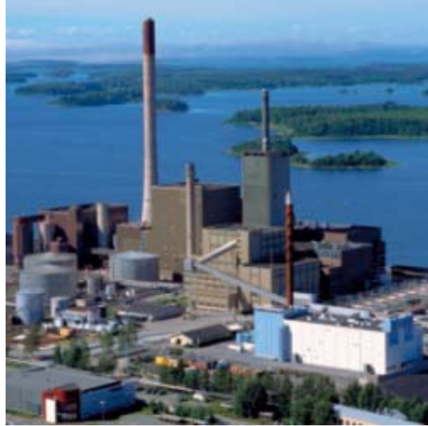
Wasa Pilot Power Plant in Vaasa.
