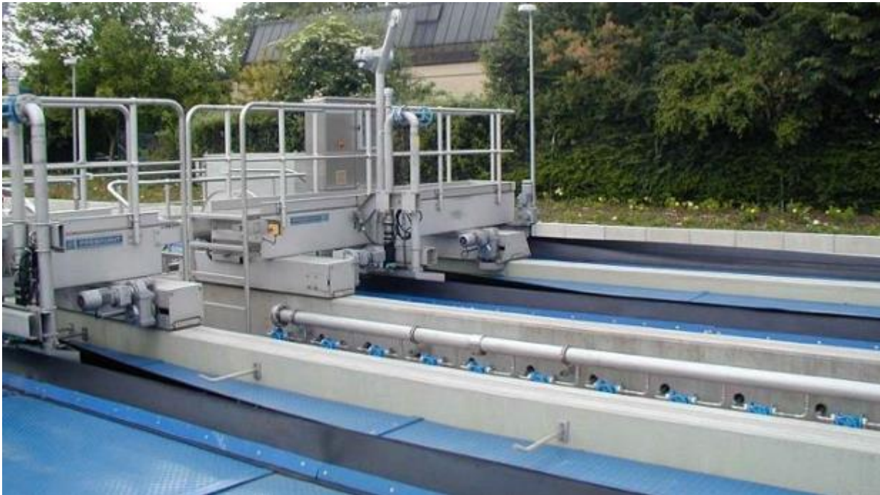
Figure 2: Example of scrapper bridge
