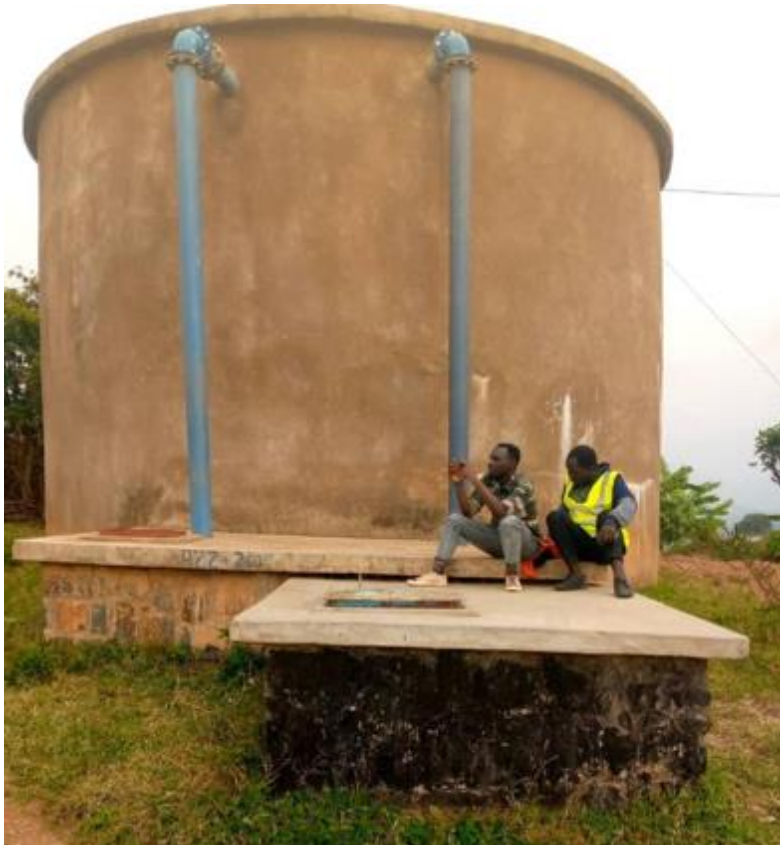
Figure 20: Existing water tank in Kibeho Sector, Nyaruguru District
