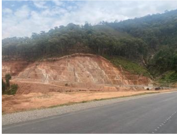
Figure 12: Unstable terrain in Nyaruguru District
