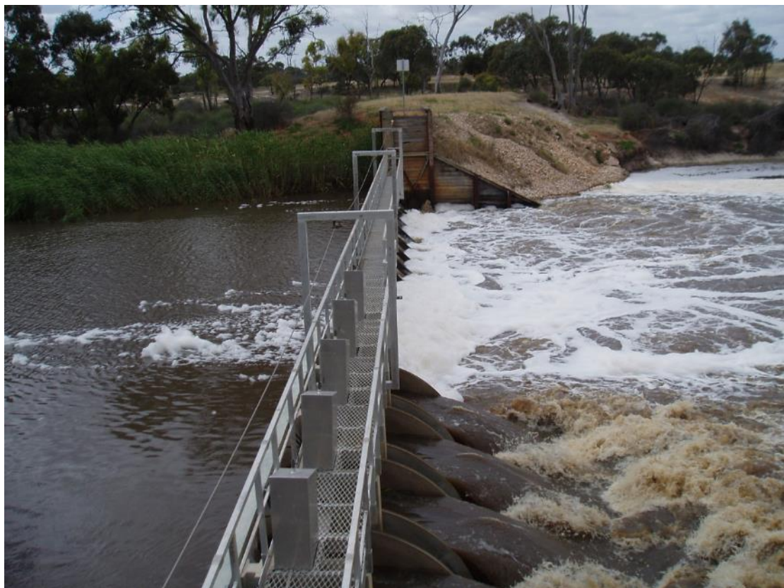
High flows through Jeparit Weir heading to Lake Hindmarsh (December 2010)
