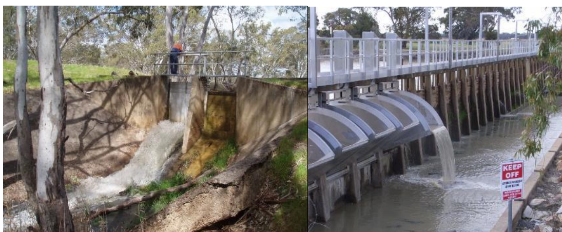
Figure 3-16. Taylor's Lake Outlet Channel Outfall (left) and the Horsham Weir (right)
