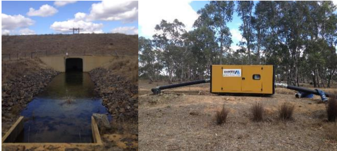
Figure 3-11. Lake Fyans Outlet Channel at Lake Fyans (left) and pumping into upper Mt William Ck refuge pool (right).
