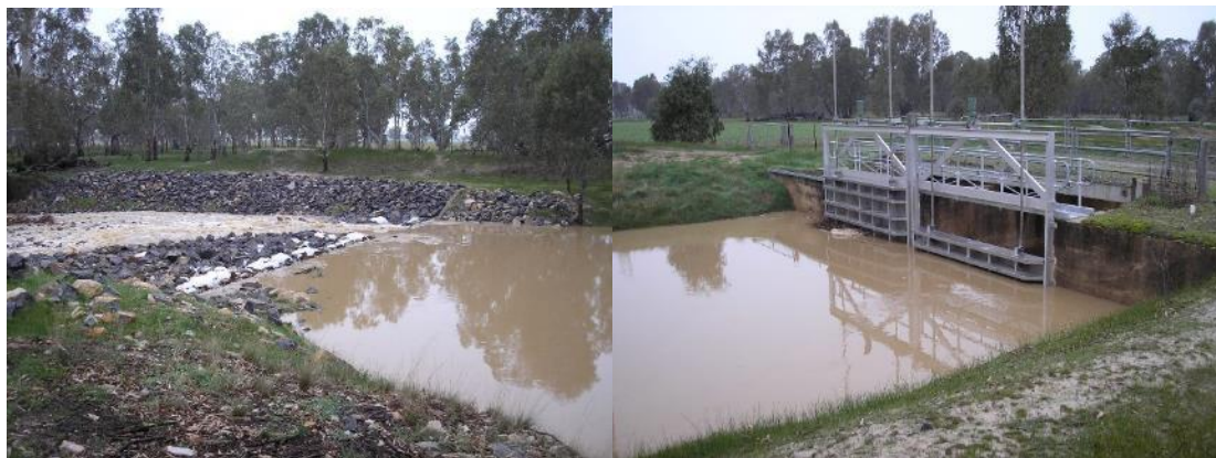
Figure 3-15. Huddleston's Weir (left) and the adjacent gates on the Wimmera Inlet Channel (right)
