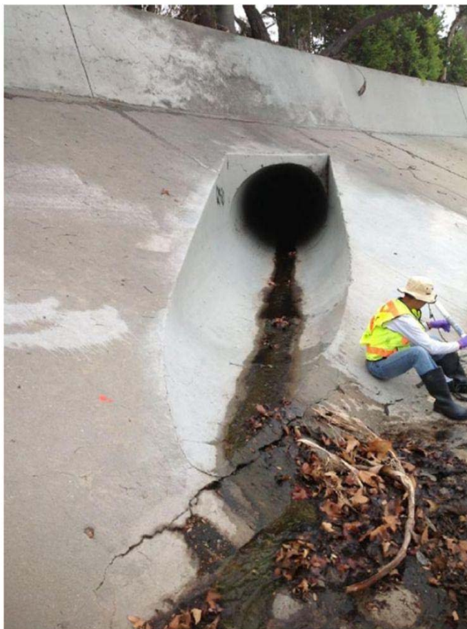
Figure 3-1 Arroyo Seco Outfall AS-17
