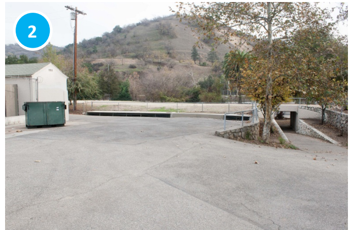
Catch basins for storm drain entering east side of park
