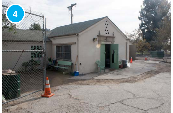
Storage area located on eastern side of park
