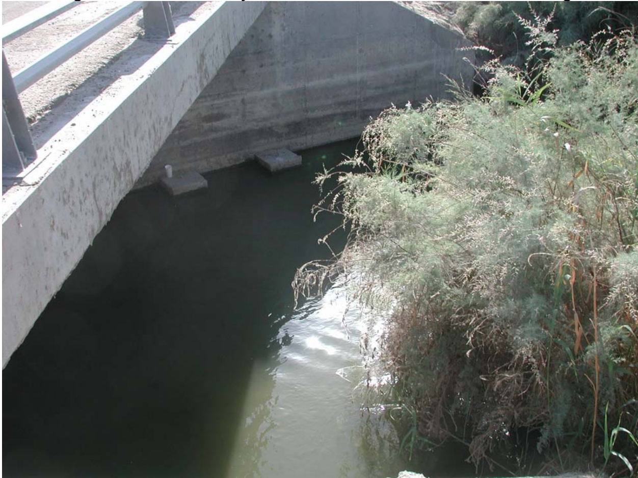
Figure 3: Coachella Valley Storm Water Channel at the Avenue 66 Bridge
