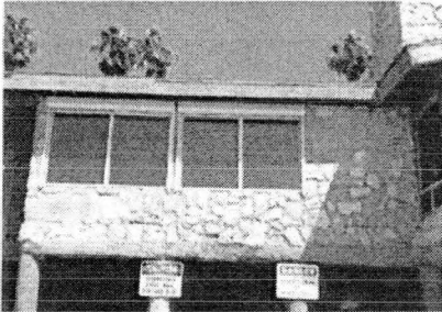
PHOTO 004 : STONE VENEER - GRID H BETWEEN 2 & 3
