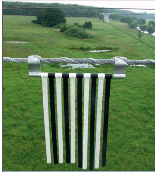
FIGURE 6.23: The RIBE line marking device is available as a swinging triangular tag or as a series of black-and-white, rigid plastic pieces that swing (pictured).
