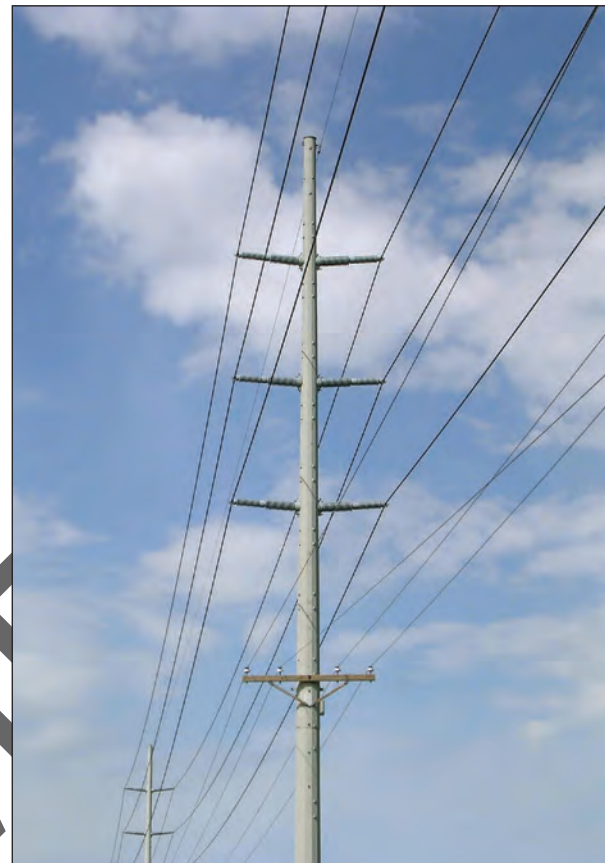
FIGURE 1.7: Distribution underbuild on a double-circuit transmission line.
