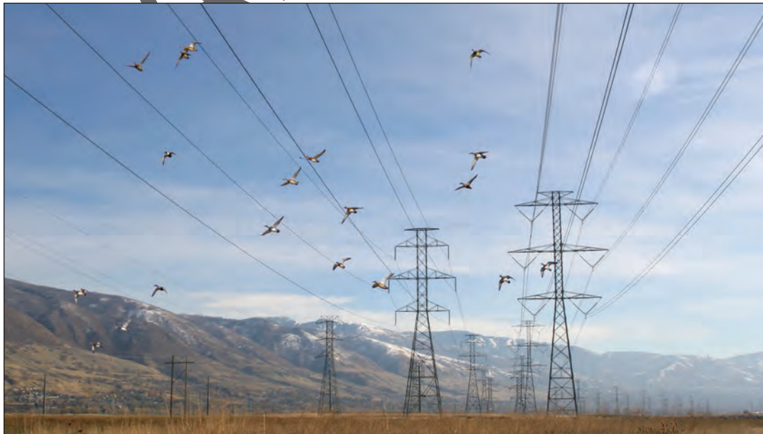
FIGURE 1.1: The highest wire on a transmission line is the shield wire, which can be difficult for birds, especially flocking birds such as waterfowl, to see.
