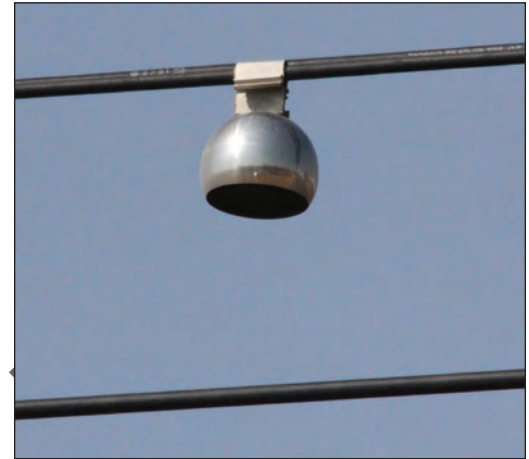
FIGURE 6.24: The Inotec BFD 88, a South African device, is a reflective stainless steel sphere reported to be visible from all angles and in low-light conditions.
