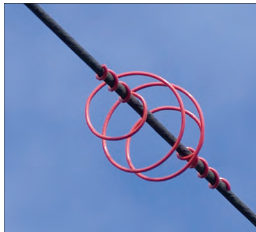
FIGURE 6.20: The Avifaune Spiral is commonly used in France and other parts of Europe.
