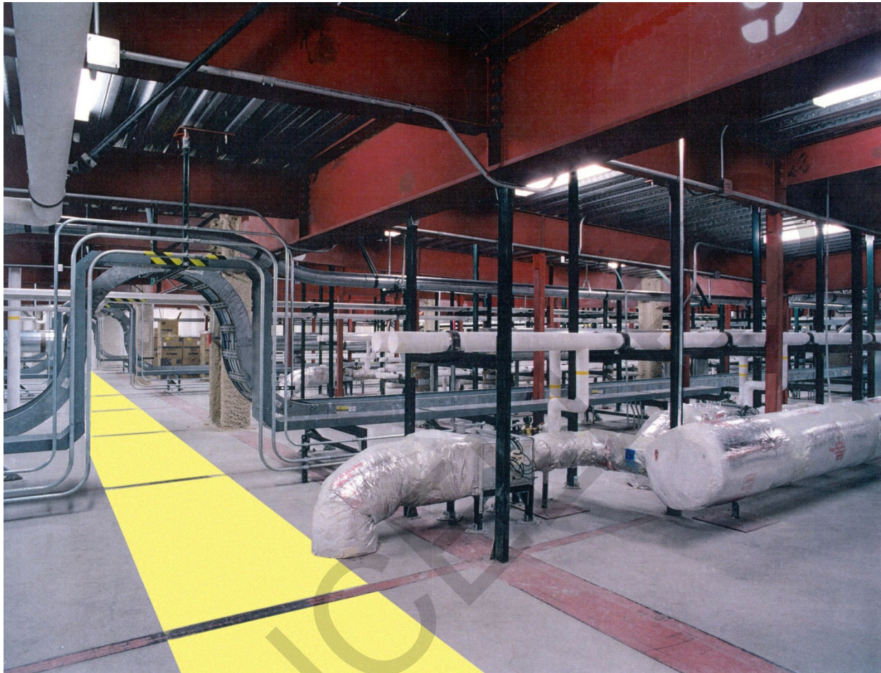
Figure E-3 Interstitial Access-Egress (Typical)
