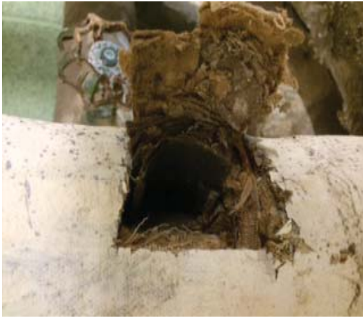
Pipe insulation with multiple layers of paper (no ACM)
