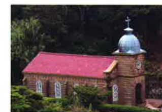
COMPONENT Kashiragashima Church (Shinkamigoto town)
