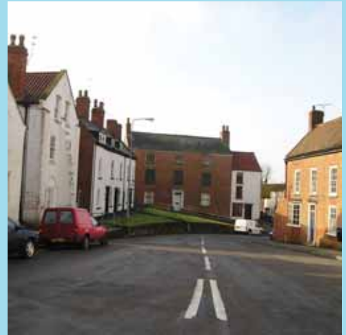
[9] View to Plough Hill showing grass bank
