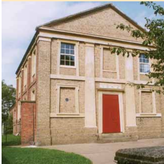
[1] Use of architectural classical orders - pilasters
