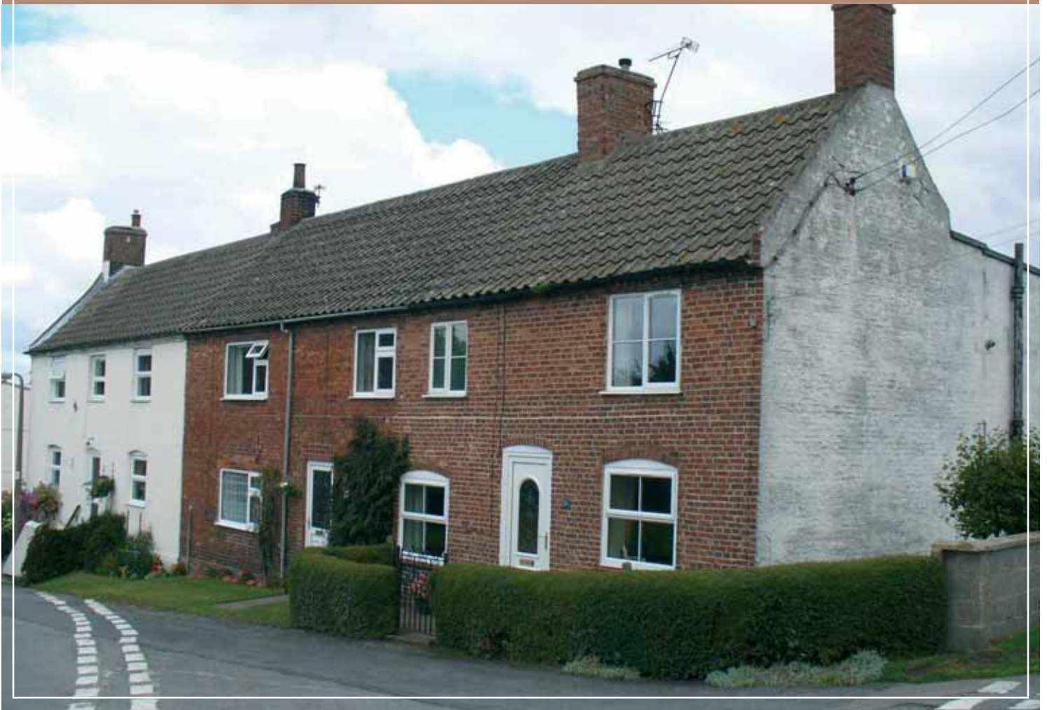
[22] North Street showing typically modest group of terraces
