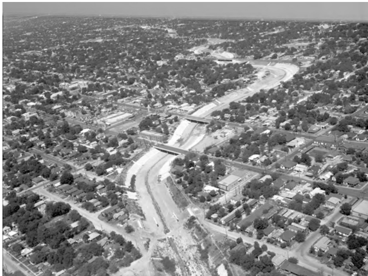
Figure 1. 1Channelization of Alazán Creek in the early 20th century
