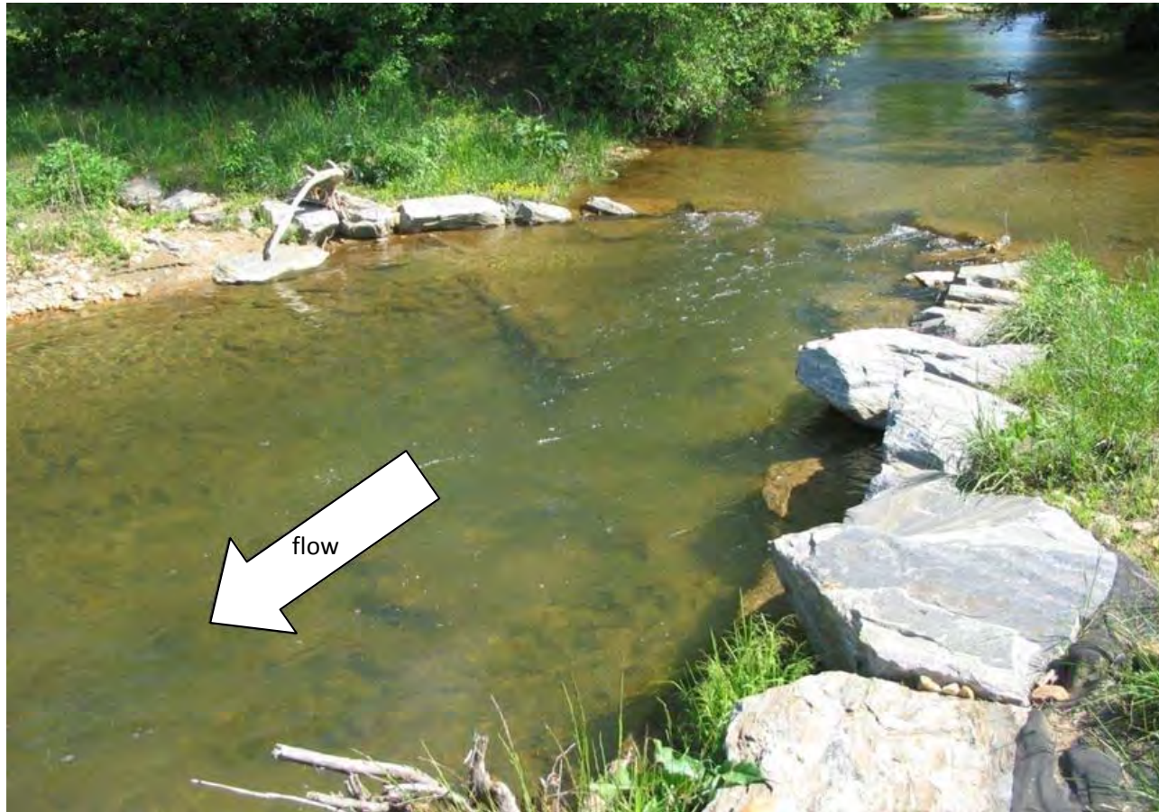
Figure 12. Photo of a Representative Functioning Rock Cross Vane
