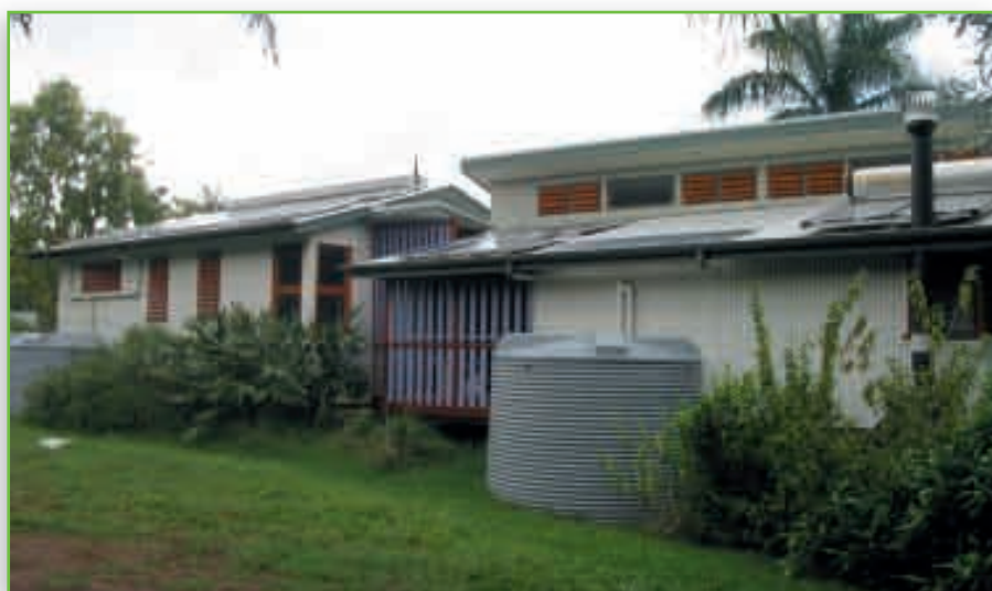
Sunbird, an energy efficient house, Cairns
