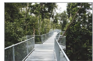
MAMU RAINFOREST CANOPY WALKWAY (PHOTO: WTMA)
