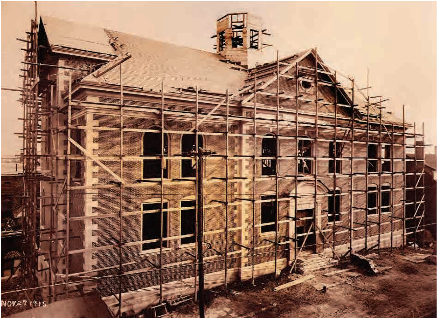
The Jonathan Bourne Whaling Museum is seen under construction in this silver gelatin print dated Nov. 27, 1915 from the Benjamin Baker Collection. The west-facing palladium windows in the rear of the Old Dartmouth Historical Society's Rogers Building are visible in the lower left corner of the photograph. NBWM 2000.100.89.3.326
