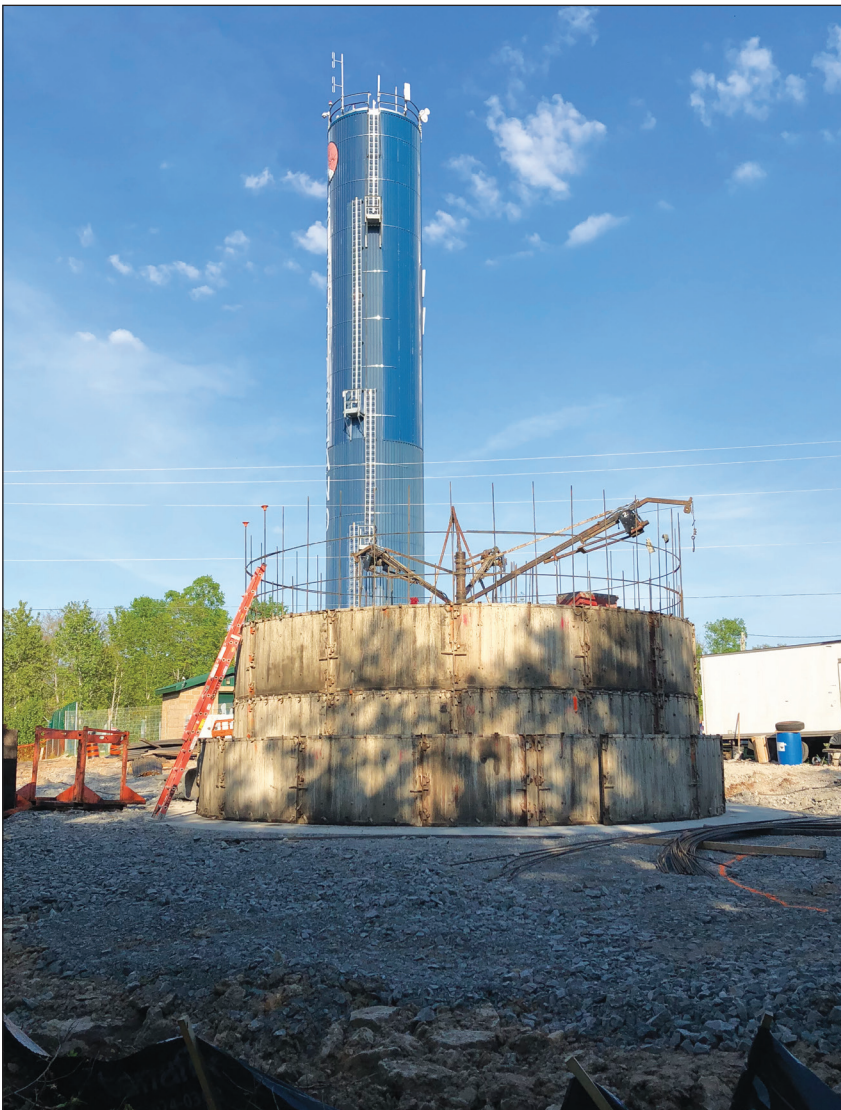
Construction of the Elevated Storage Reservoir is progressing nicely.
