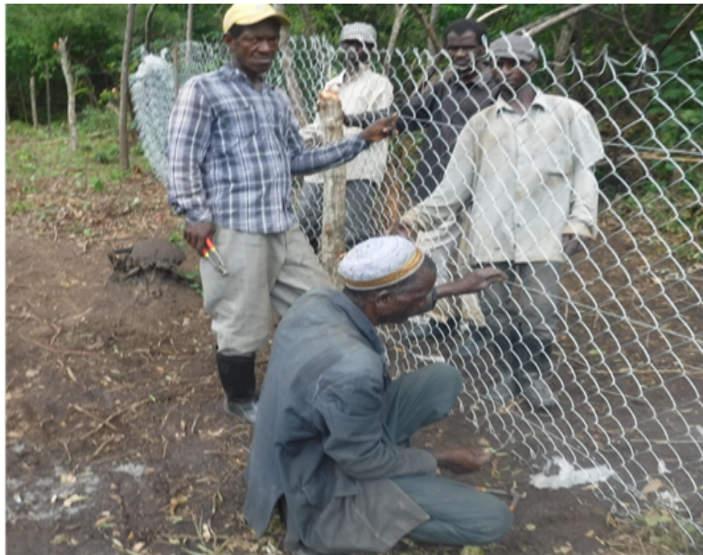
Figure 44. Installation of fencing
