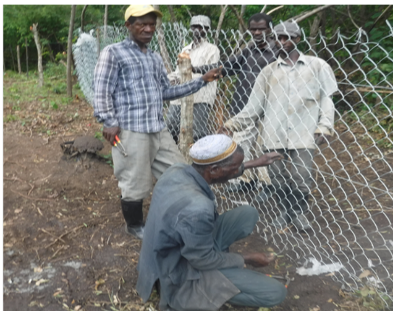
Figure 44 : Installation des grillages
