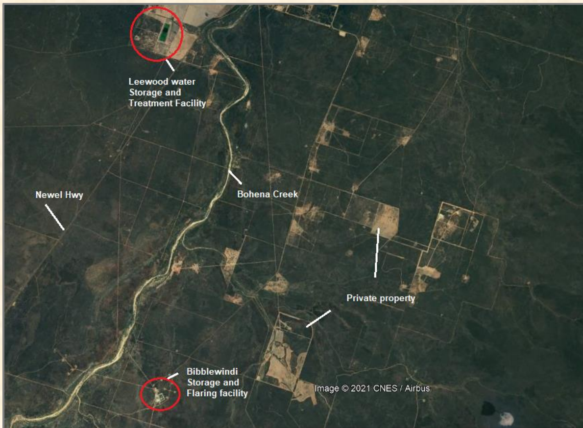
Current gasfield infrastructure in the forest (From CNES / Airbus 2021)
