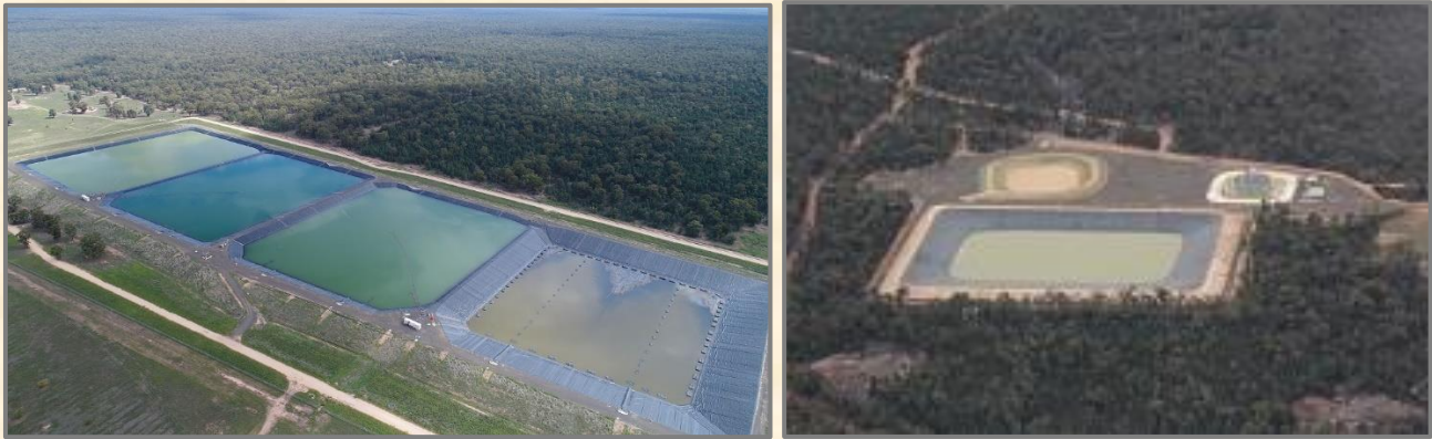
Left: Leewood holding ponds. Right: Bibblewindi facility.
