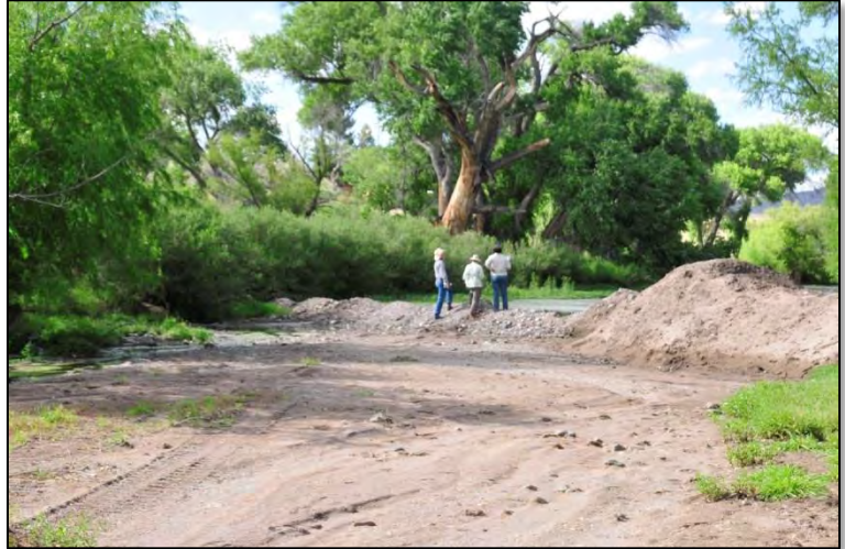
Figure 10. Earthen irrigation dam in the river channel looking upstream and north.
