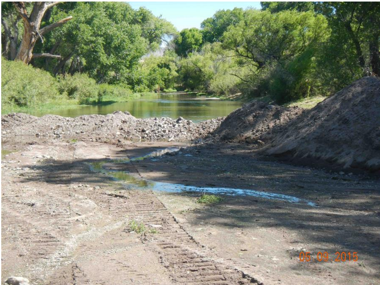
Figure 5. Mimbres River diversion dam (K. Gadzia)
