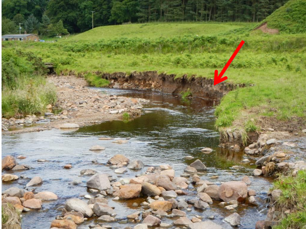
Picture 4. The foreground of this picture is the location of a recently dug pool that has filled in with material from upstream. This is primarily because the pool was over wide and deep, and effectively acting as a silt trap. The rock weir created at the tail of the pool also exacerbated this and is likely to have increased erosion around the weir. Also note the increased erosion upstream in the centre of shot (arrowed), resulting from the bed material upstream moving downstream to fill the void created by the pool.
