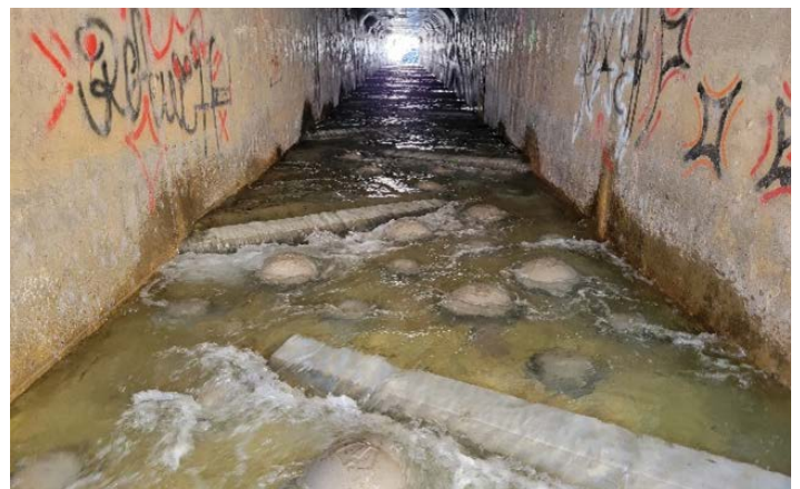
Figure 7. Baffles and hemispheres after being installed in the Canyon Creek culvert under Interstate 70.
