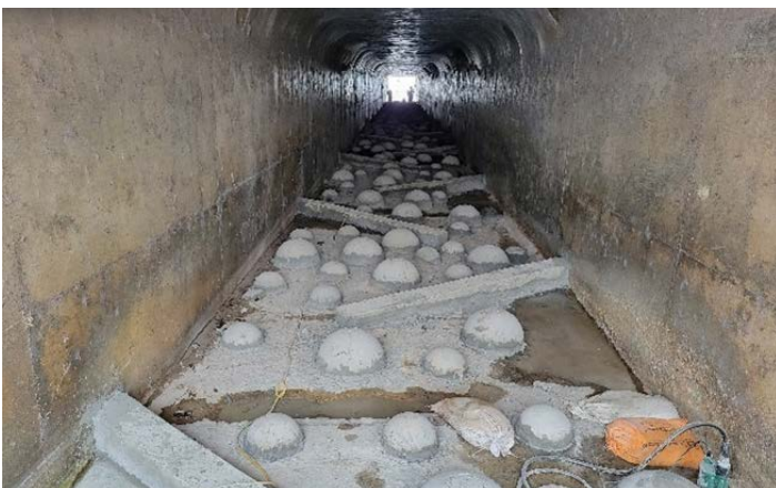
Figure 7. Baffles and hemispheres after being installed in the Canyon Creek culvert under Interstate 70.
