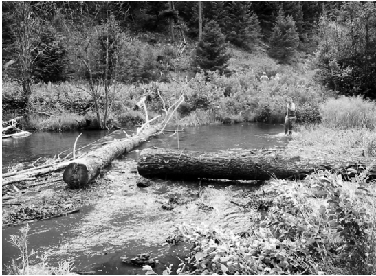
Figure 3. Whole trees being placed in Belmont Creek. Note cable (indicated by arrow) attached to log and via tackle (behind shrubs in background) draft horses.
