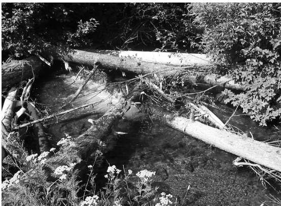
Figure 4. Representative structure site on Belmont Creek illustrating juxtaposition of tree pieces in order to fragment currents at high flows. Note that some tree pieces are completely above the stream surface, which is typical during times of lower flow.
