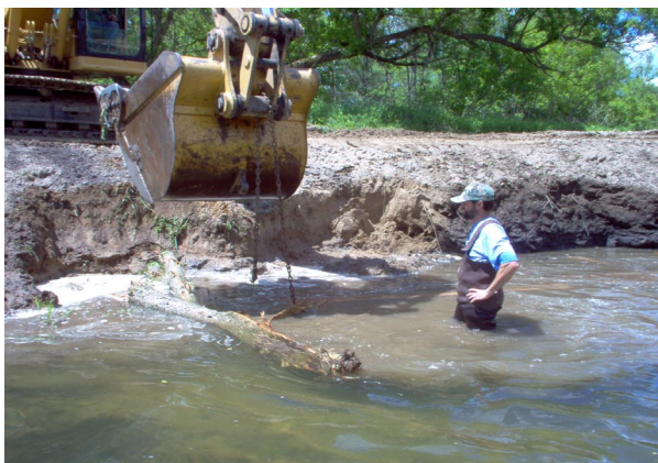
Figure 3. Anchoring woody debris
