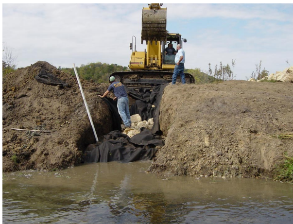
Figure 5. Hibernaculum placed in streambank under rock riprap.
