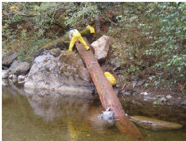
Figure 5. Wood and Rock Instream Structures Austin Creek, Russian River, Sonoma County, California
