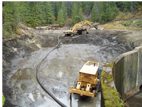
Figure 4. Excavation of sediment stored behind Cedar Creek Dam (Inter-fluve, Inc. photo)
