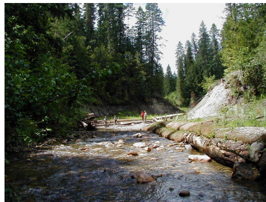
Figures 1 and 2. Cedar Creek Dam before (top) and after removal (bottom) in October 2005.
