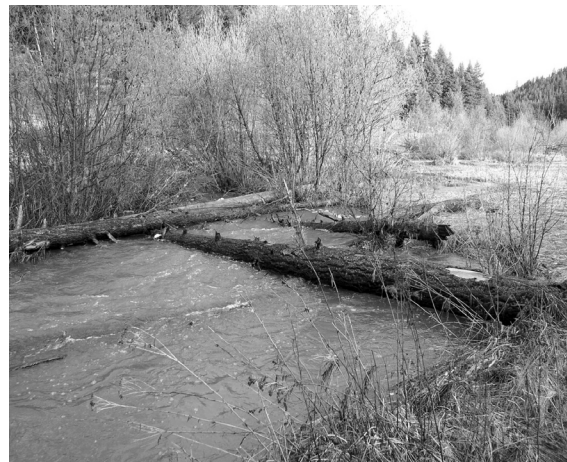
Figure 5. Placed tree pieces during Belmont Creek’s high flow, when channel-forming action is greatest.
