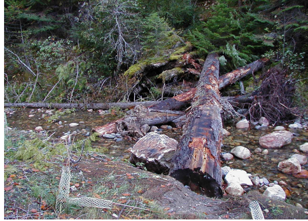
Figure 9. Channel spanning log jams were installed to increase gravel deposition.
